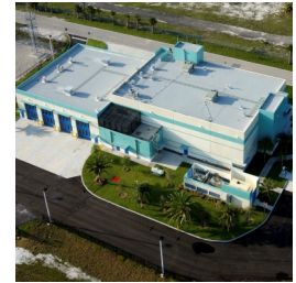
Fort Lauderdale Emergency Operations Center
