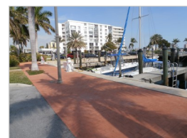
Seawall Remediation at Lake Harbor Park Marina
