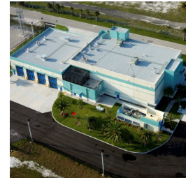
Fort Lauderdale Emergency Operations Center
