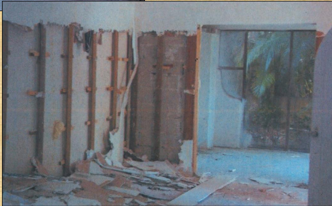
Enclosed Porch - Before
