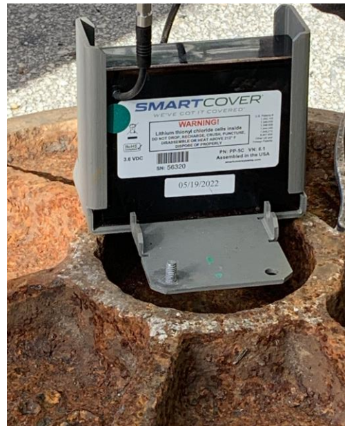
Smart Covers predict sewer overflows
