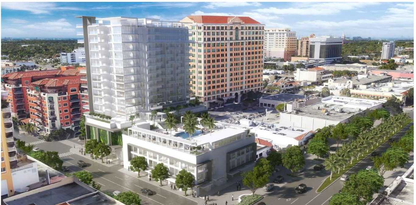
Proposed project and existing conditions
