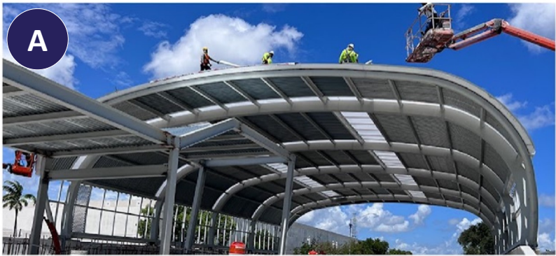
A South Corridor: Bus Transit, under construction
