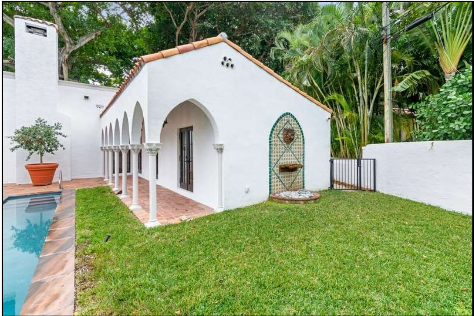
North (Rear) Façade – After
