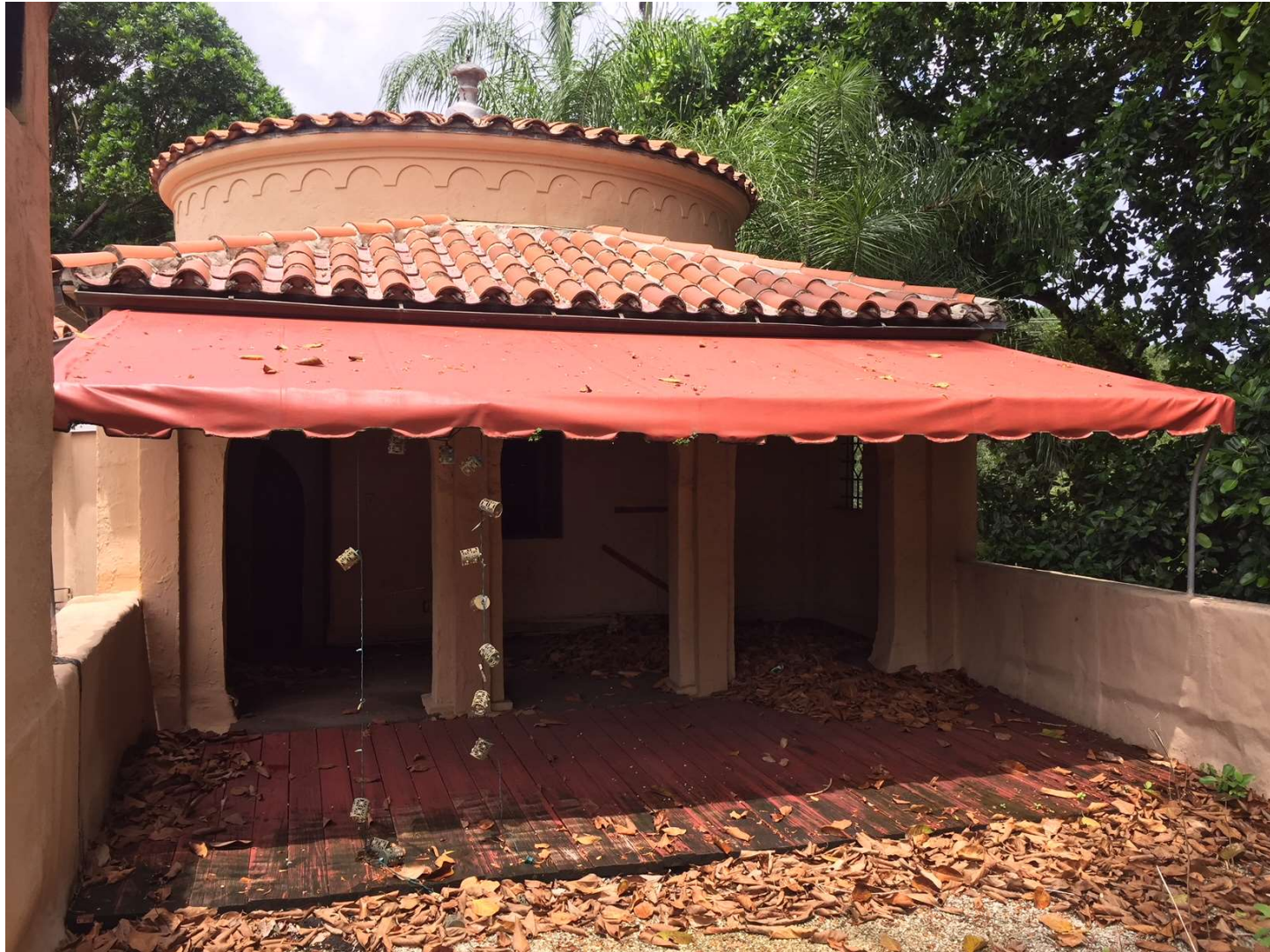
Second Floor Roof Terrace (looking east) – Before
