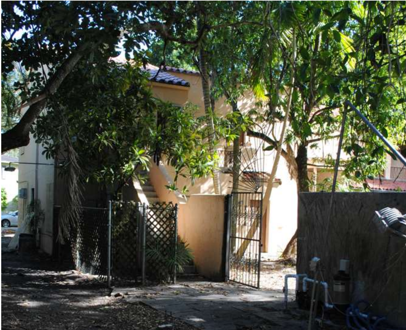
Northwest Corner – Before
