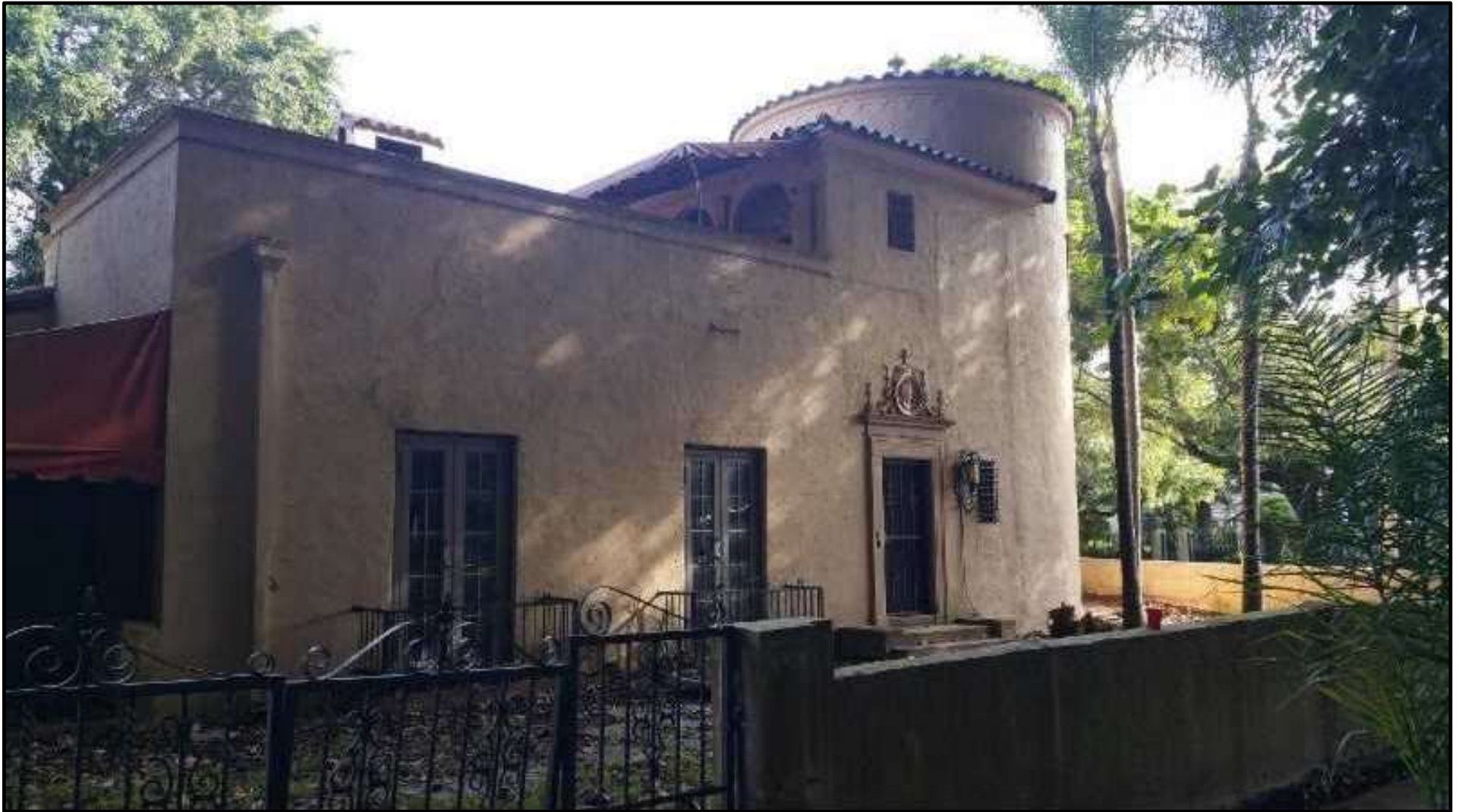
South (Front) Façade - Before
