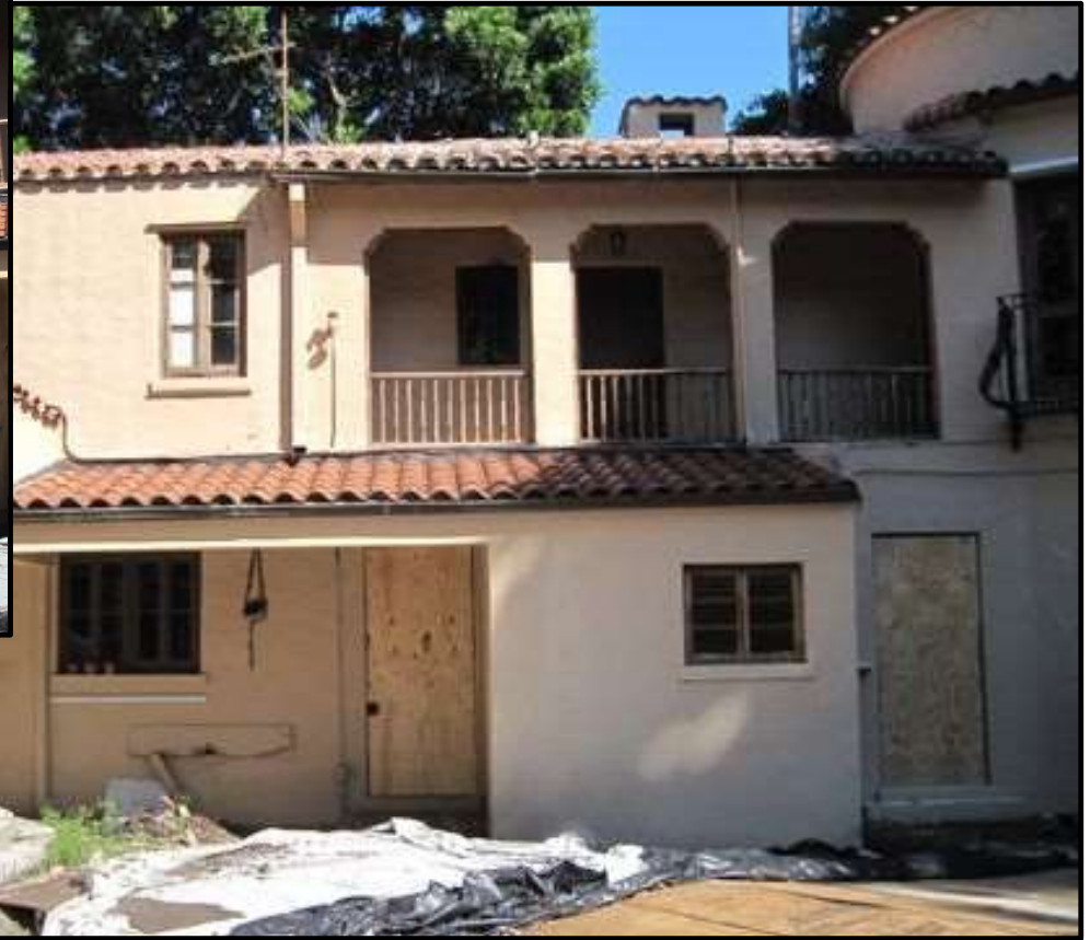
West (Rear) Facade – Before
