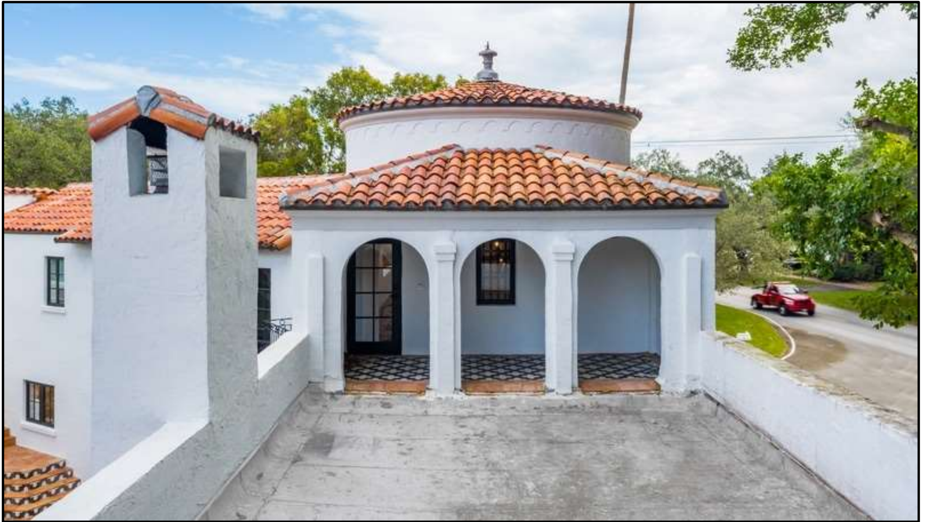
Second Floor Roof Terrace (looking east) – After
