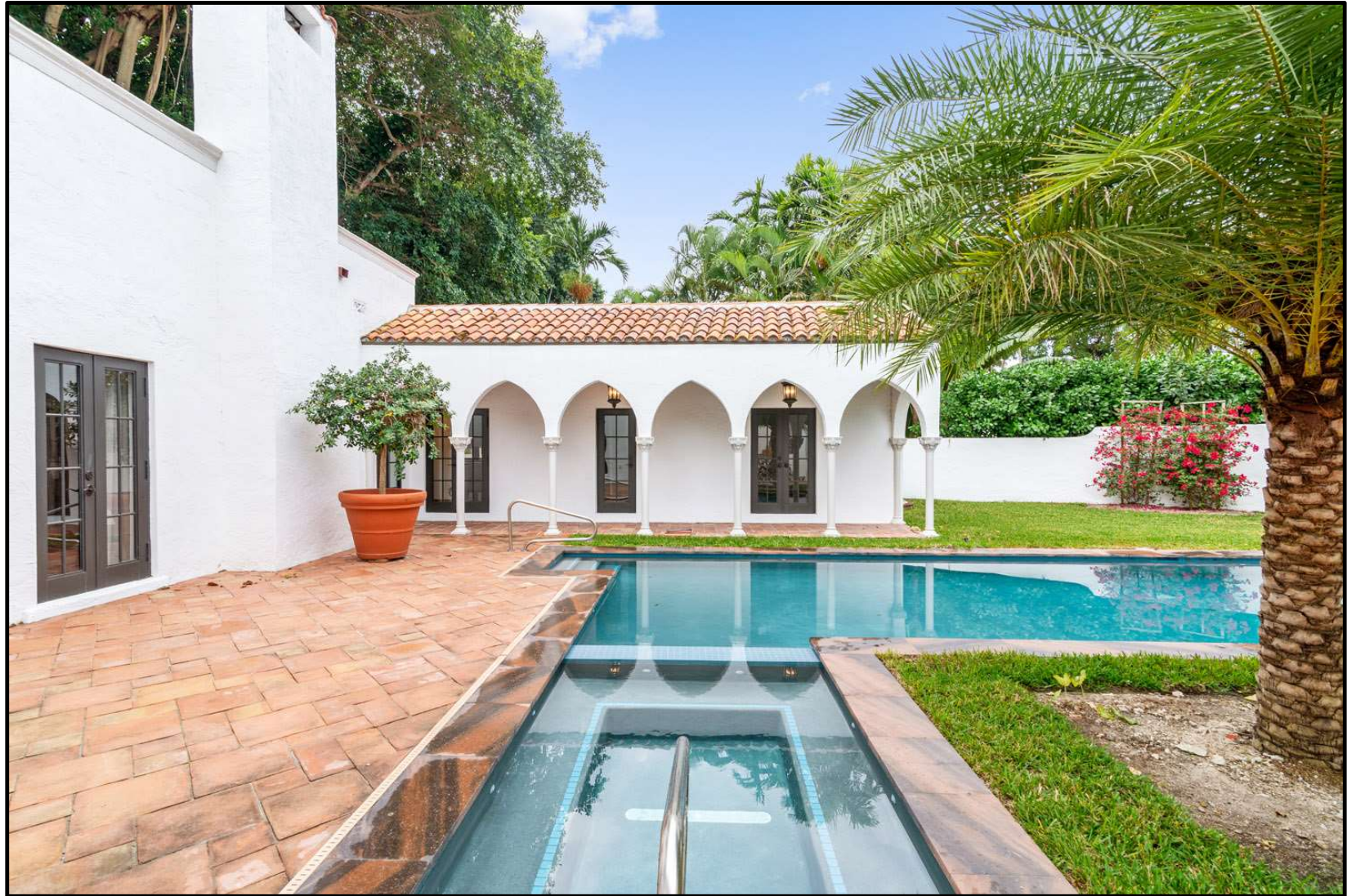
East (Rear) Façade – After
