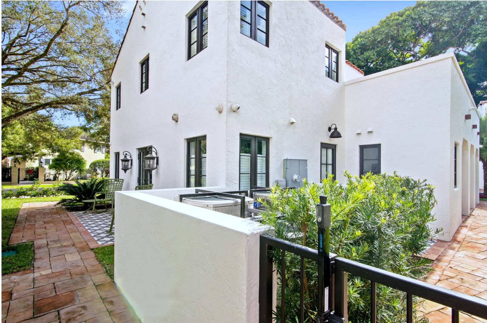
Northwest Corner – After
