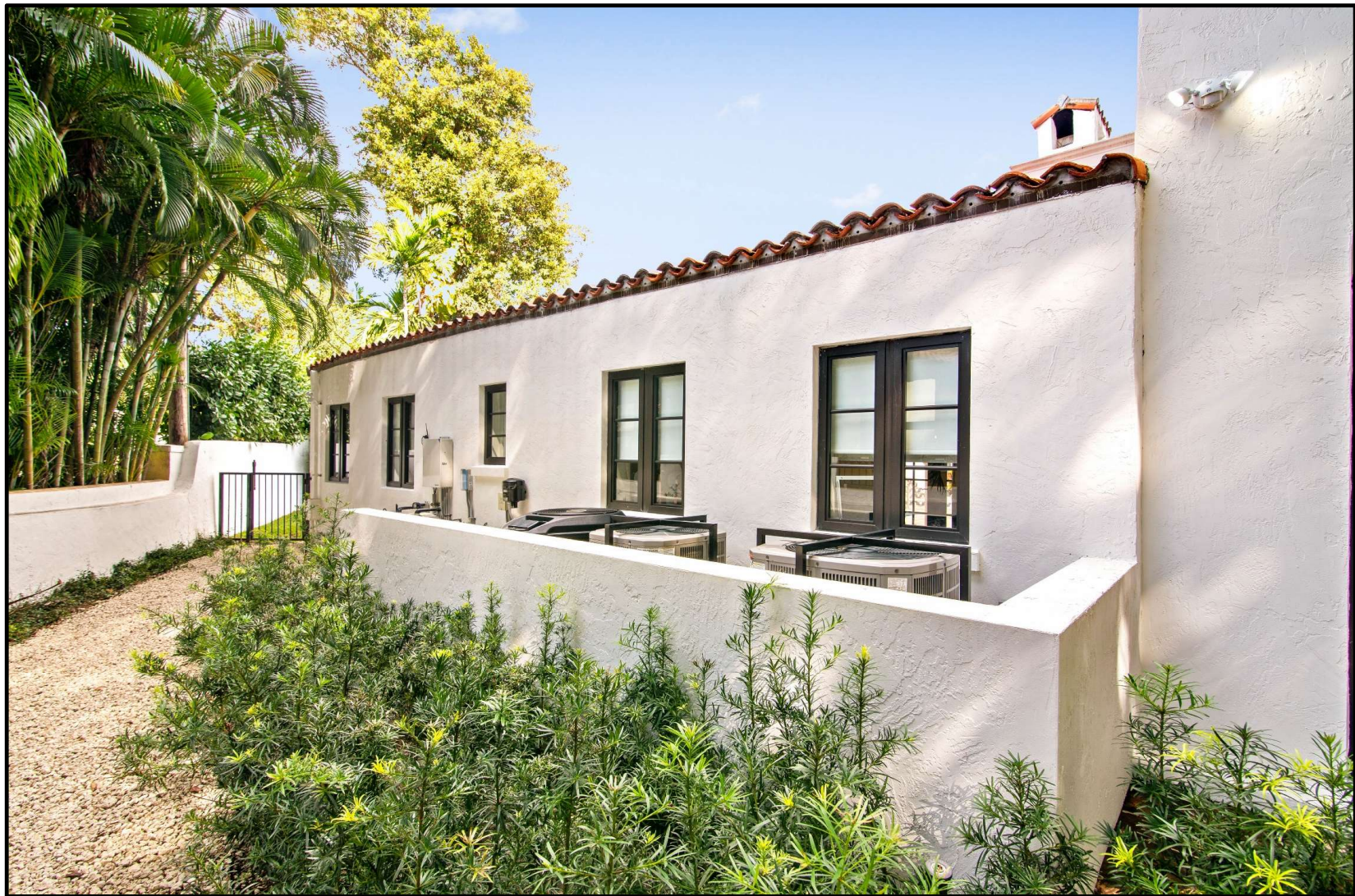
West Façade – After
