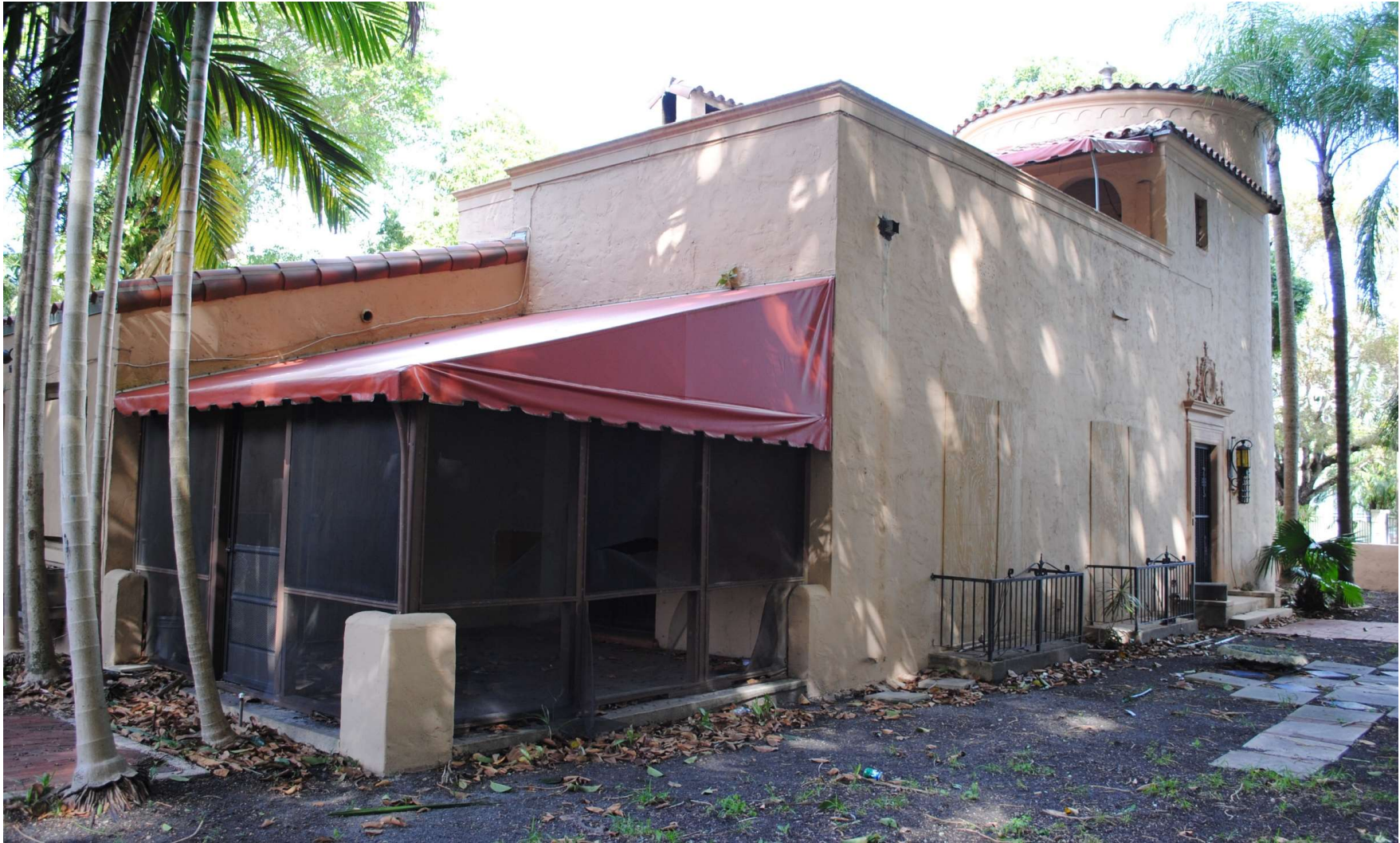
South (Front) Façade - Before
