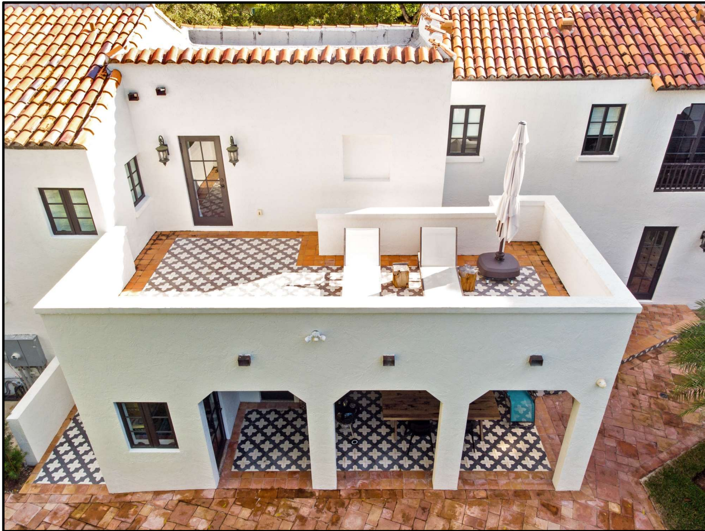
West (Rear) Facade – After
