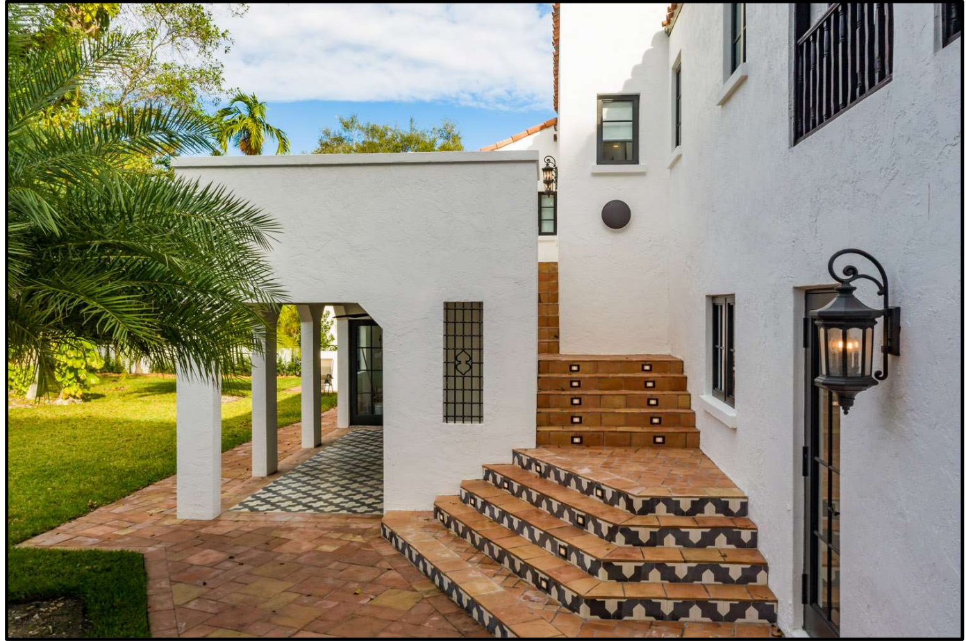
West Façade (looking north) – Before & After
