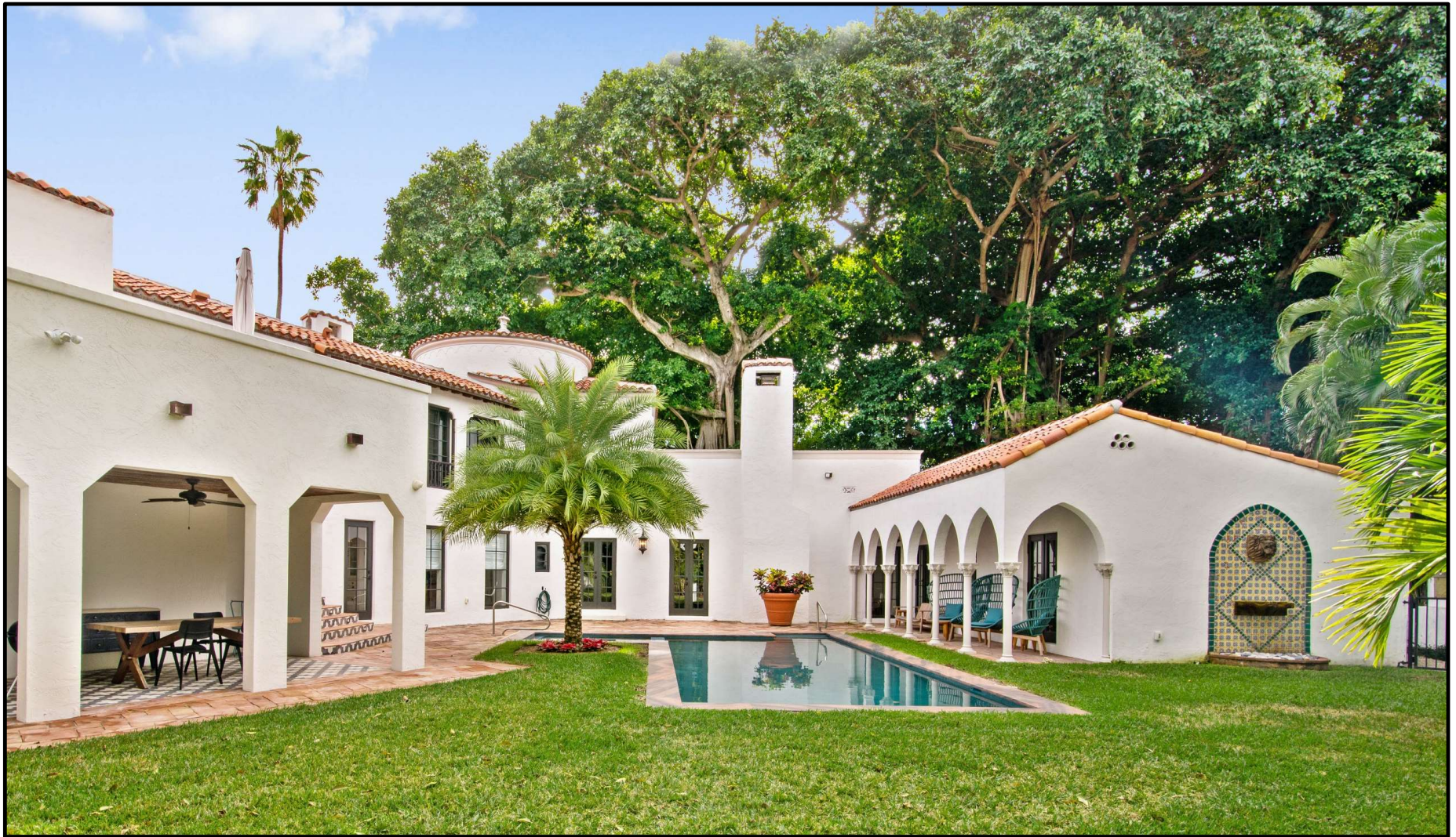
West and North (Rear) Facades – After
