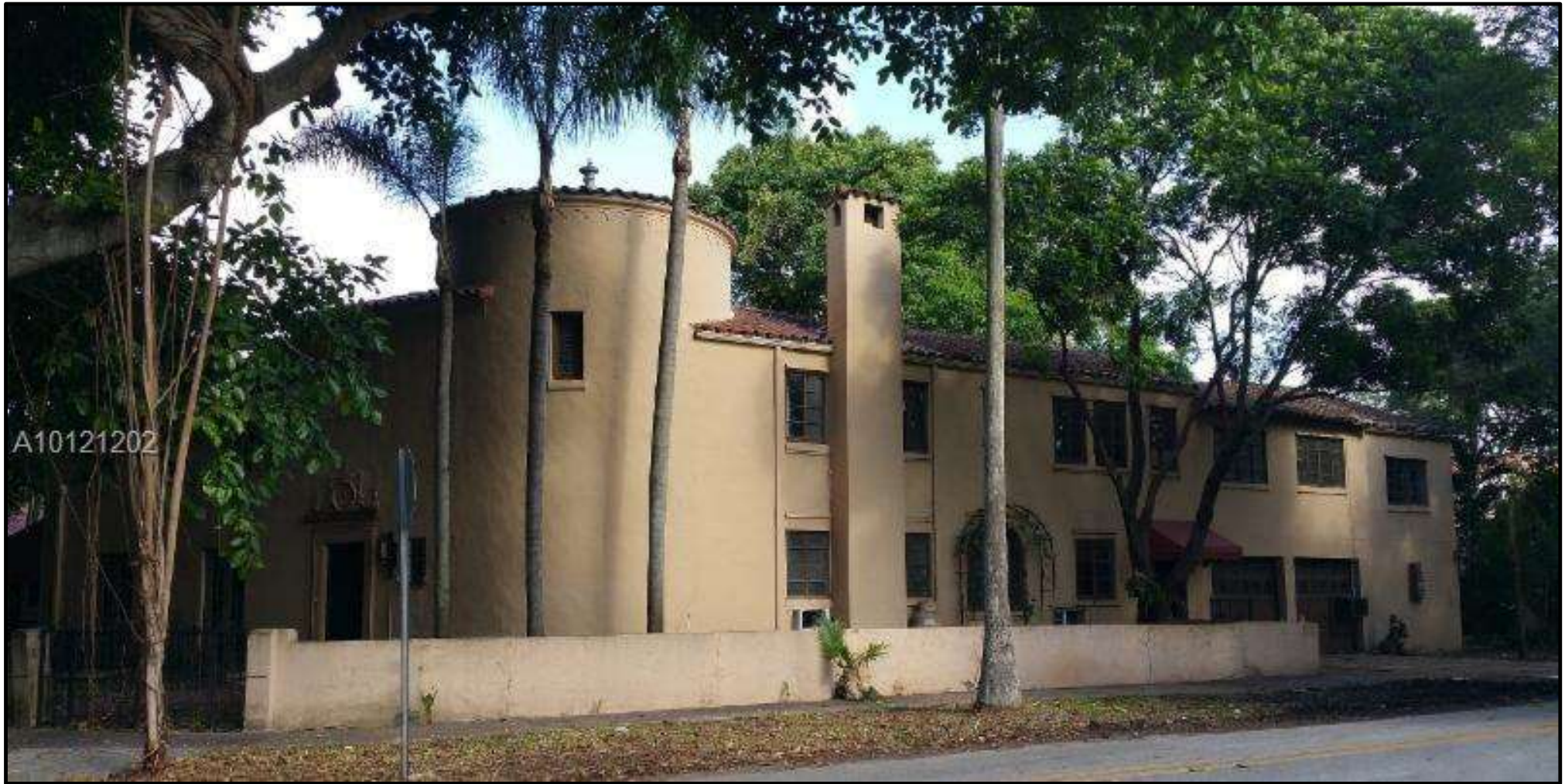
East Façade – Before
