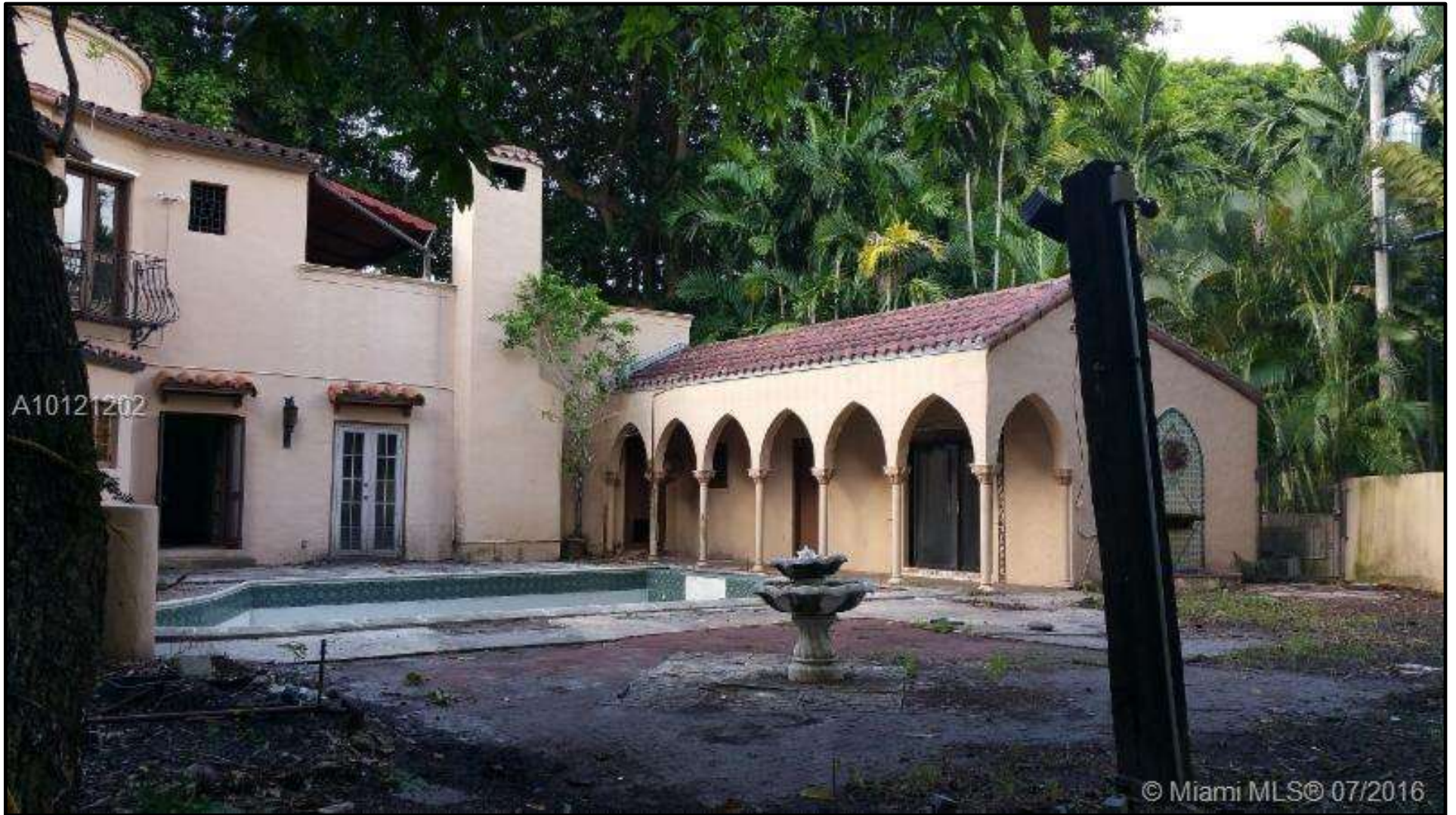
North and East (Rear) Façades – Before
