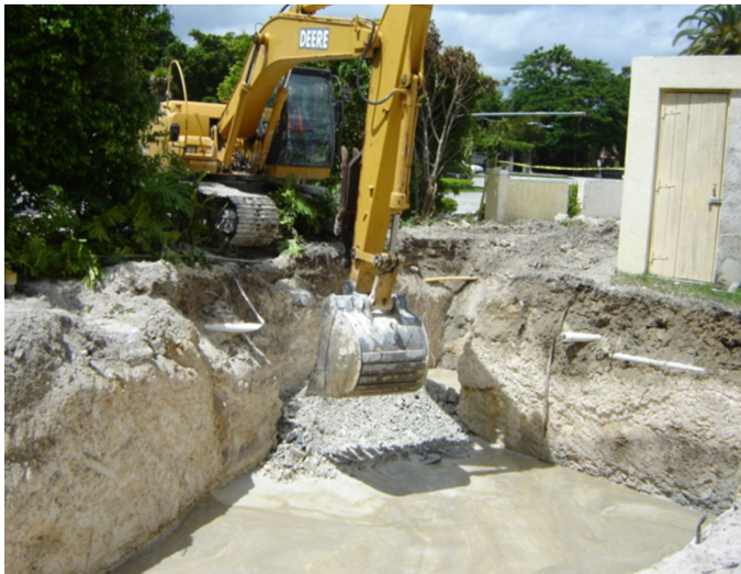
Coral Gables Country Club Remediation Source Removal
