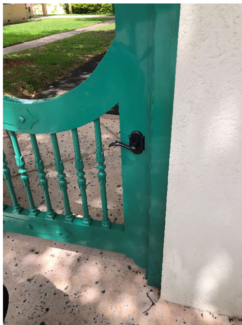
Auto-close gate with handle installed at street ends
