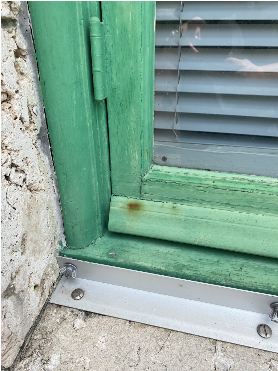
Exterior Window Detail (West Elevation)
