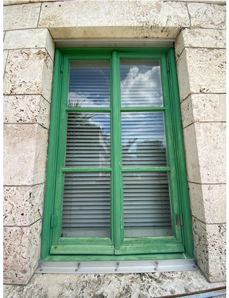
Exterior Window (West Elevation)
