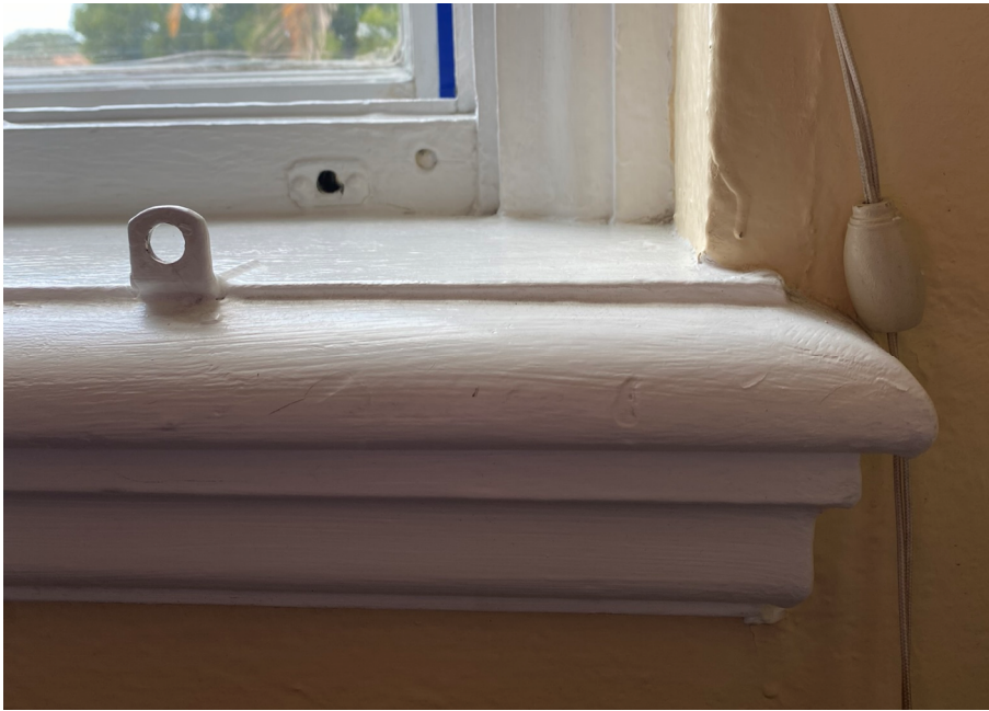
Interior Window Detail (West Elevation)
