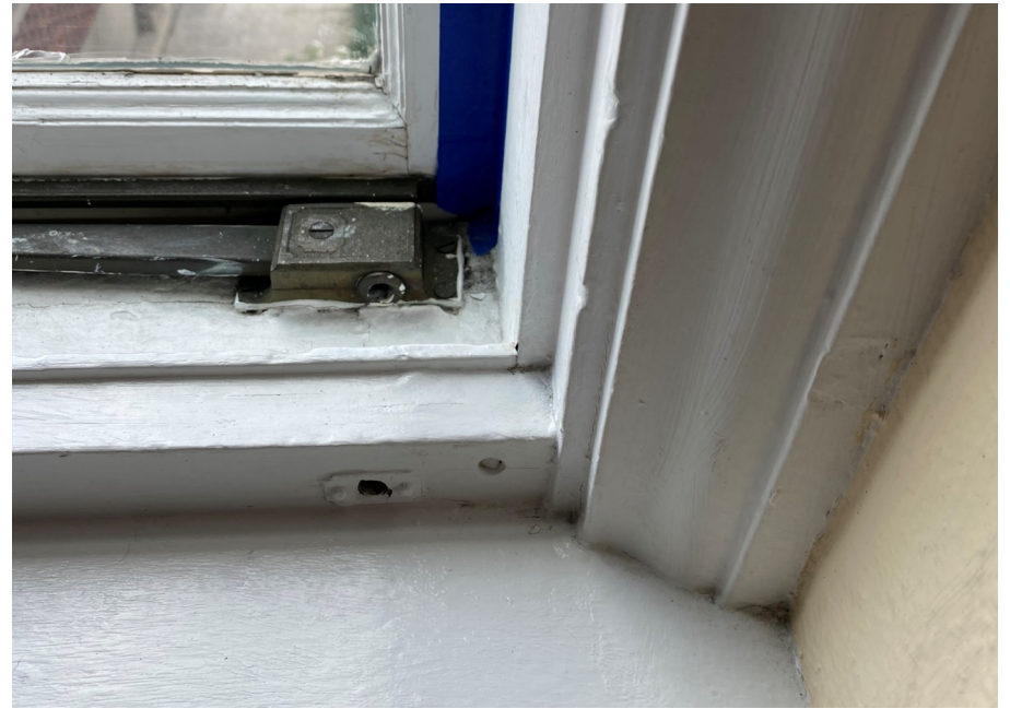
Interior Window Detail (West Elevation)
