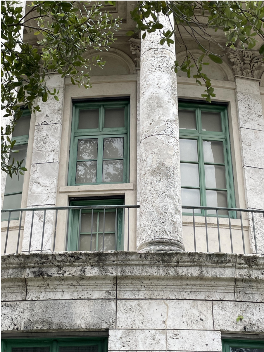
Exterior Windows (East Elevation)
