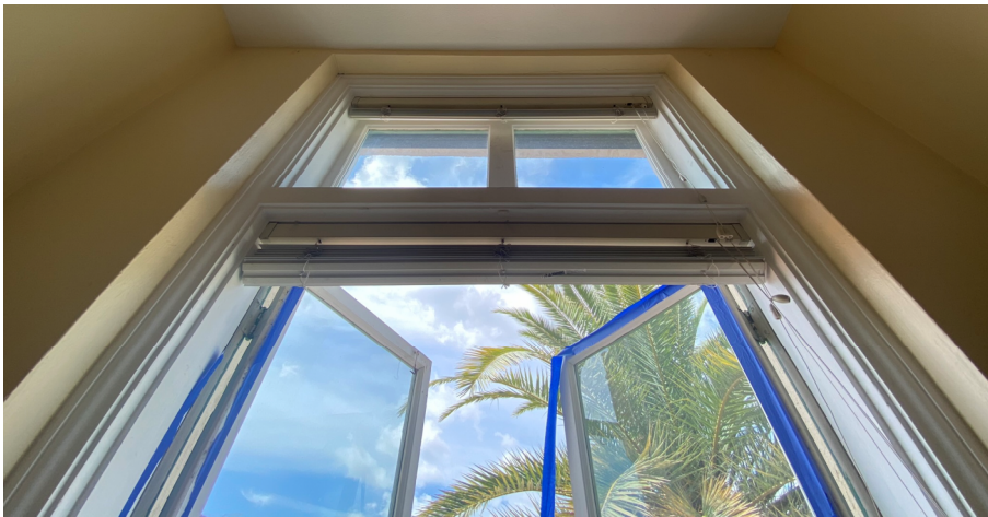
Interior Window (West Elevation)
