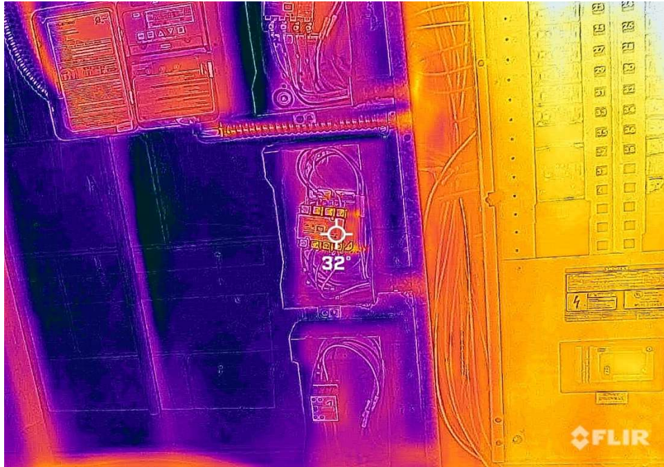
Item 28: Relay at 32.0 Degrees Celsius (delta 2.0C)
