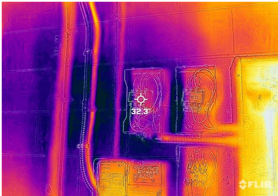
Item 33: Relay at 32.3 Degrees Celsius (delta 2.3C)
