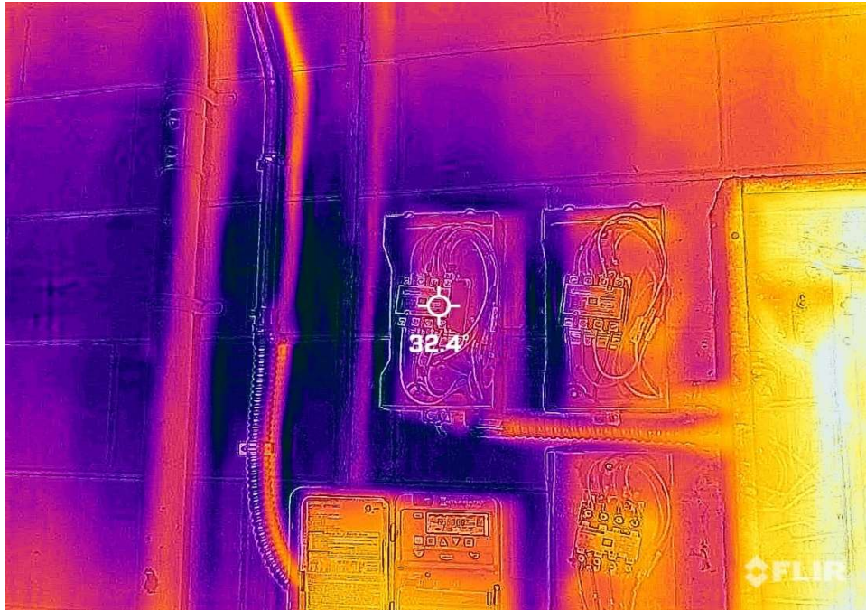
Item 34: Relay at 32.4 Degrees Celsius (delta 2.4C)
