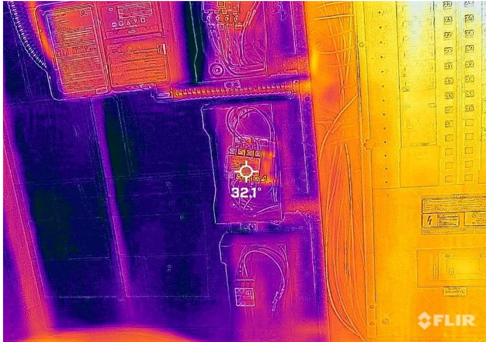
Item 32: Relay at 32.1 Degrees Celsius (delta 2.1C)
