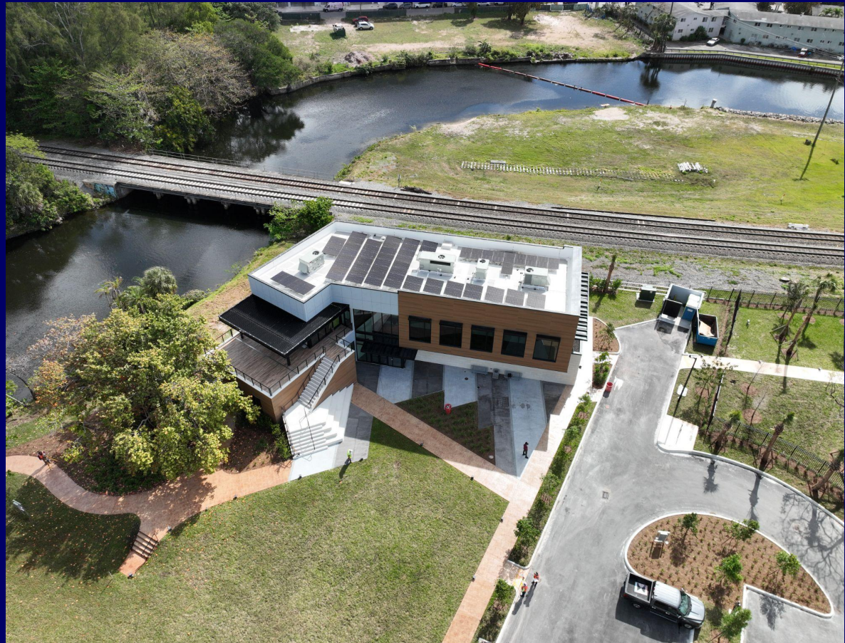
New, nearly 8,000-sf wildlife hospital and education center that is nearly complete.
