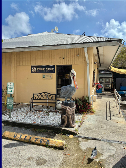
Current 950-sf building built by Miami-Dade County for PHSS in 1992
