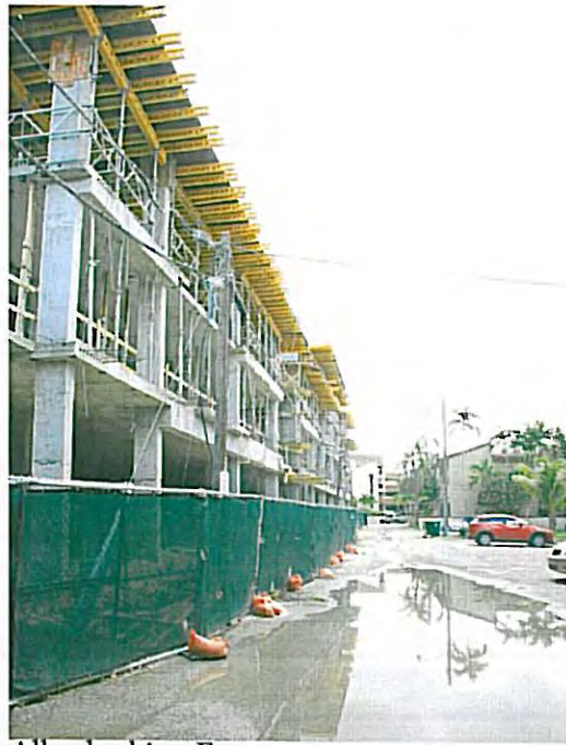
Alley looking East
