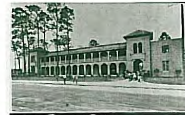
Coral Gables Elementary Continuous Open Loggia with Chained Structure and concrete balcony & barrel the roof
