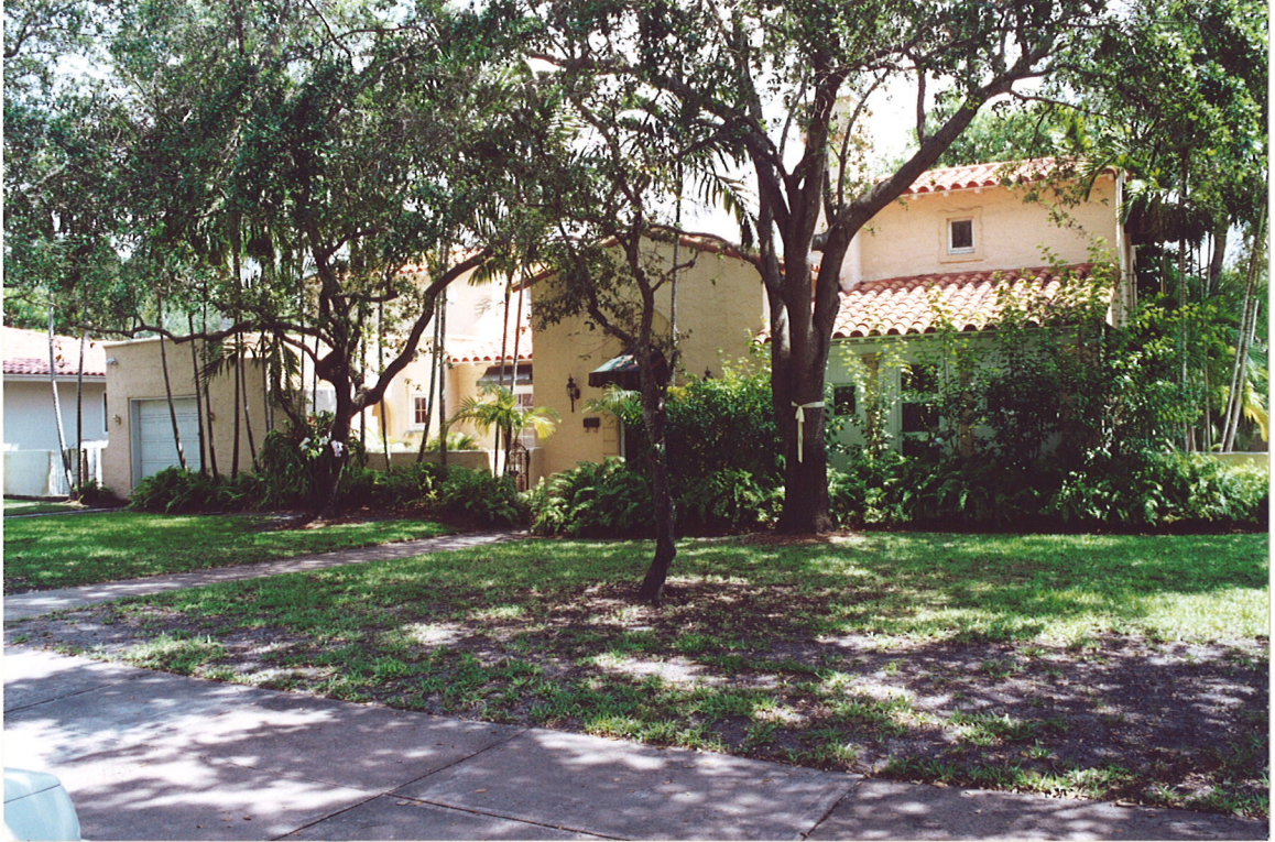
PHOTO #4—West (Front) Elevation (View from Country Club Prado)
