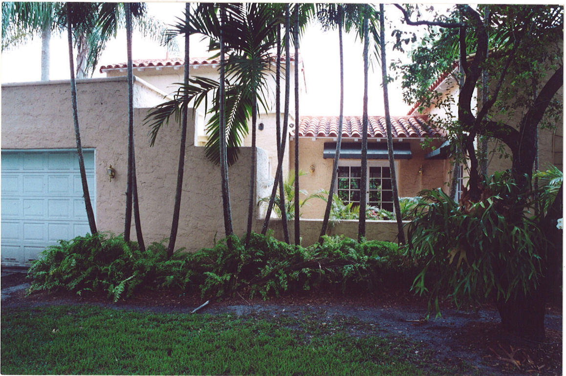
PHOTO #5—West (Front) Elevation (Exist. Courtyard)
