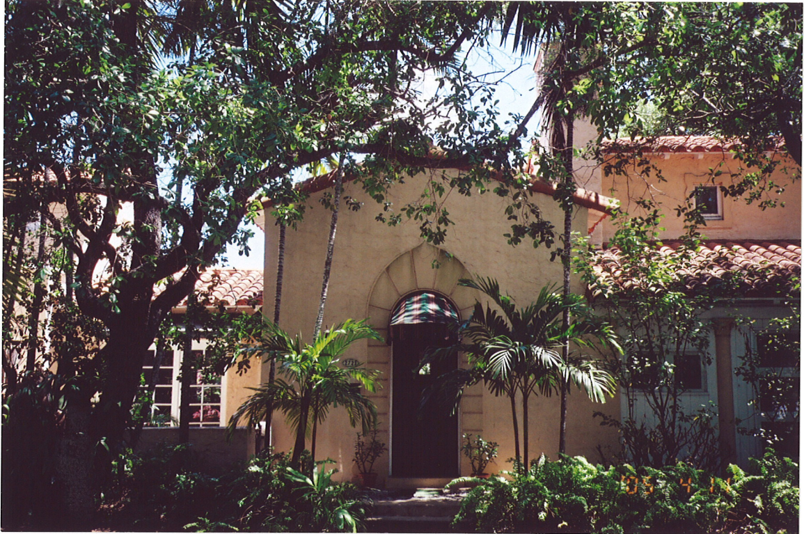
PHOTO #6—West (Front) Elevation (Main Entrance)
