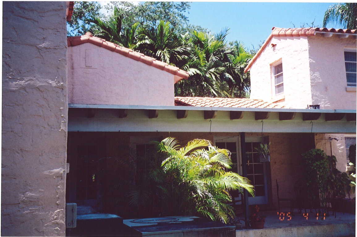
PHOTO #2—East (Rear) Elevation (Exist. Covered Terrace-View 2)
