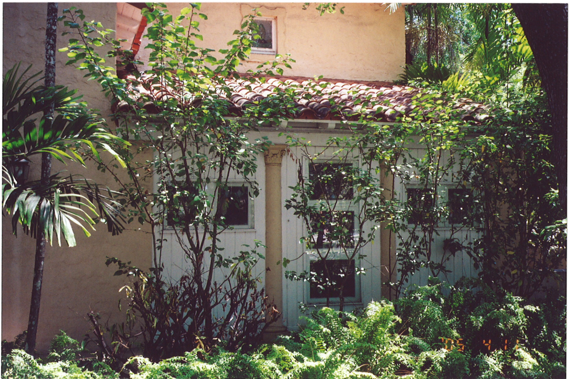
PHOTO #7—West (Front) Elevation (Front Terrace)
