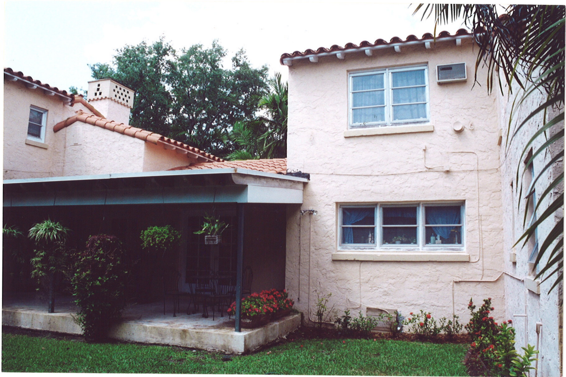
PHOTO #1—East (Rear) Elevation (Exist. Covered Terrace-View 1)
