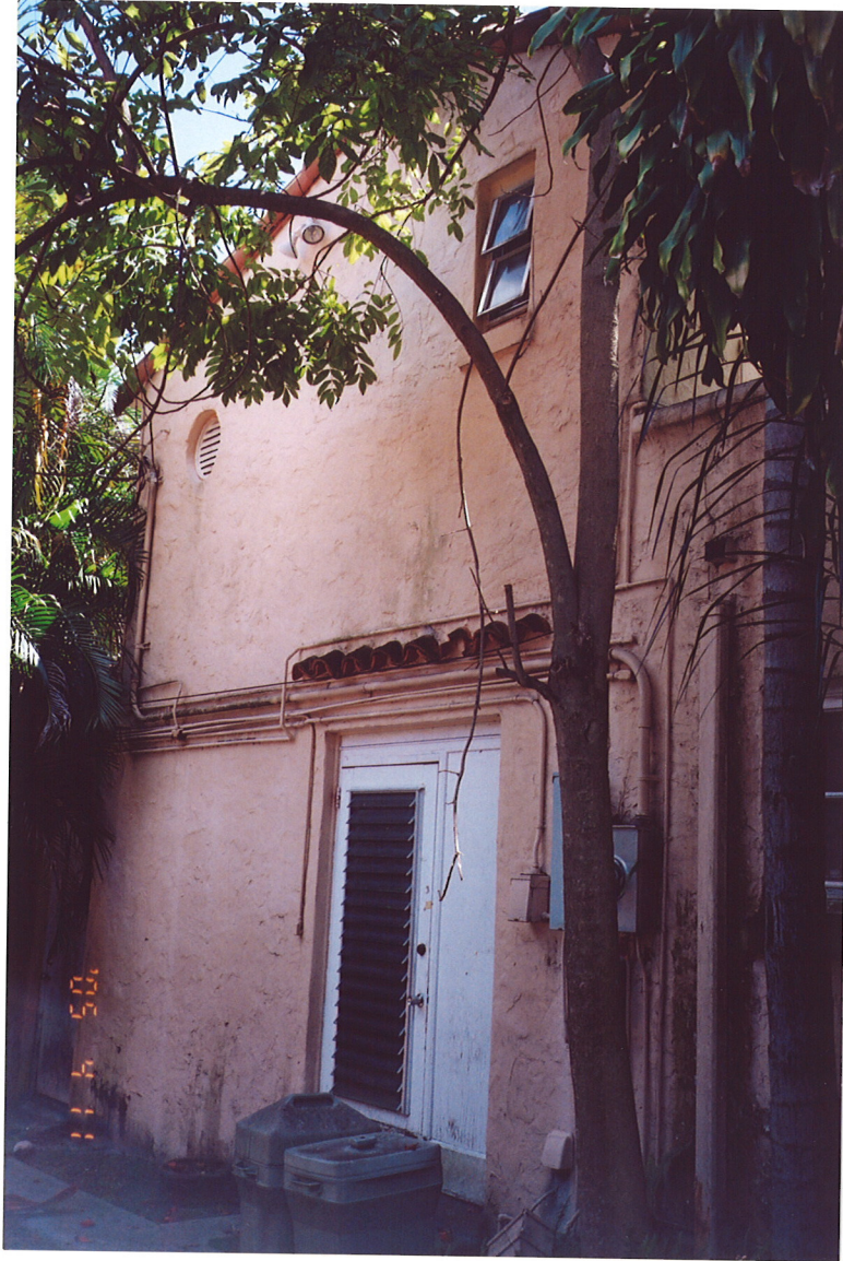
PHOTO #9—North (Side-Interior) Elevation (Exist. Door to Laundry Room)
