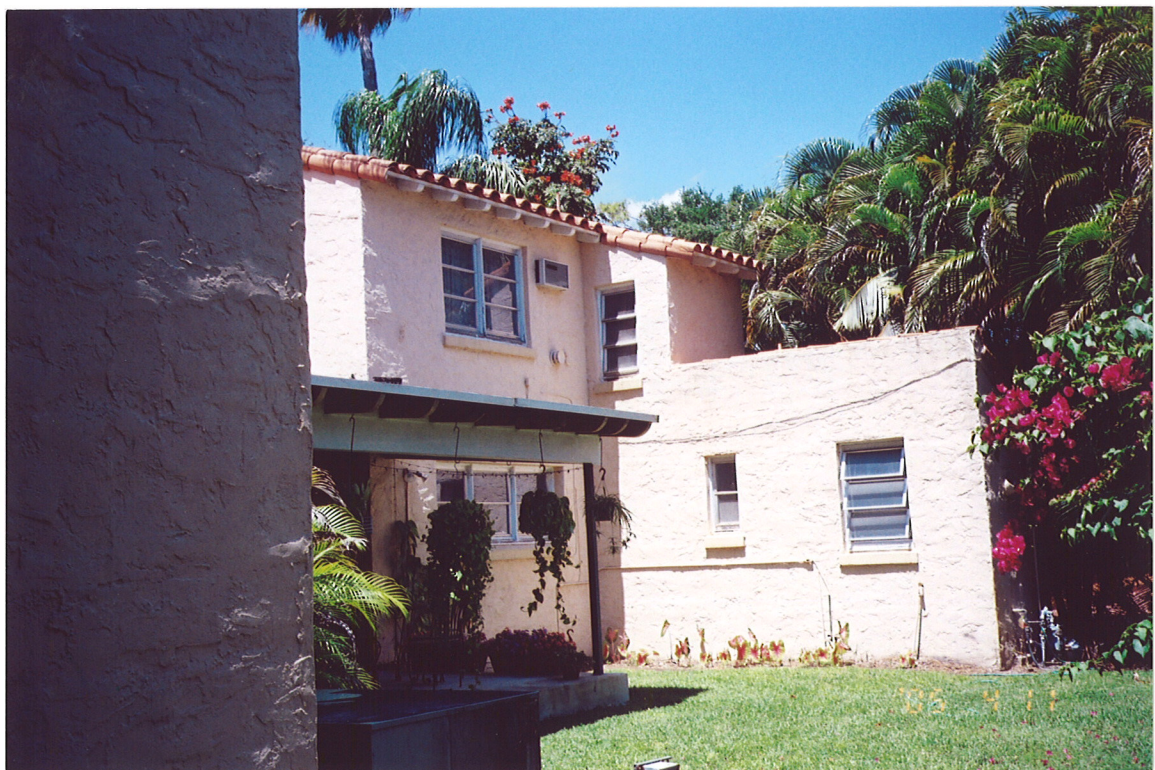
PHOTO #15— Existing Rear Yard (View of location of proposed Open Terrace)
