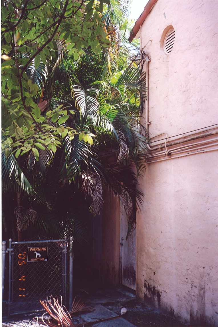
PHOTO #8—North (Side-Interior) Elevation (Exist. Doors to Utility Rooms)
