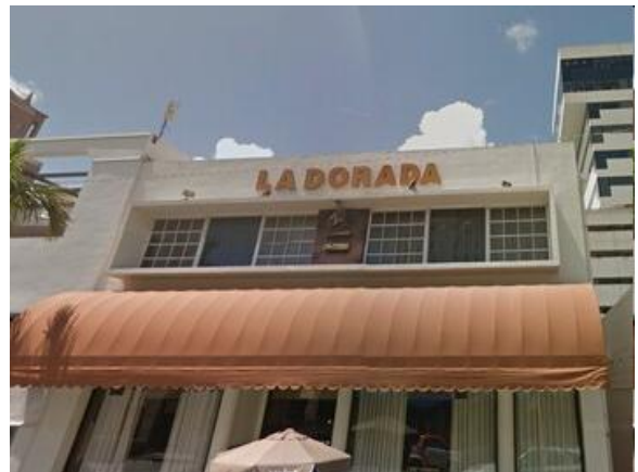
Lease 6 Giralda Plaza Pedestrian Mall Retail
