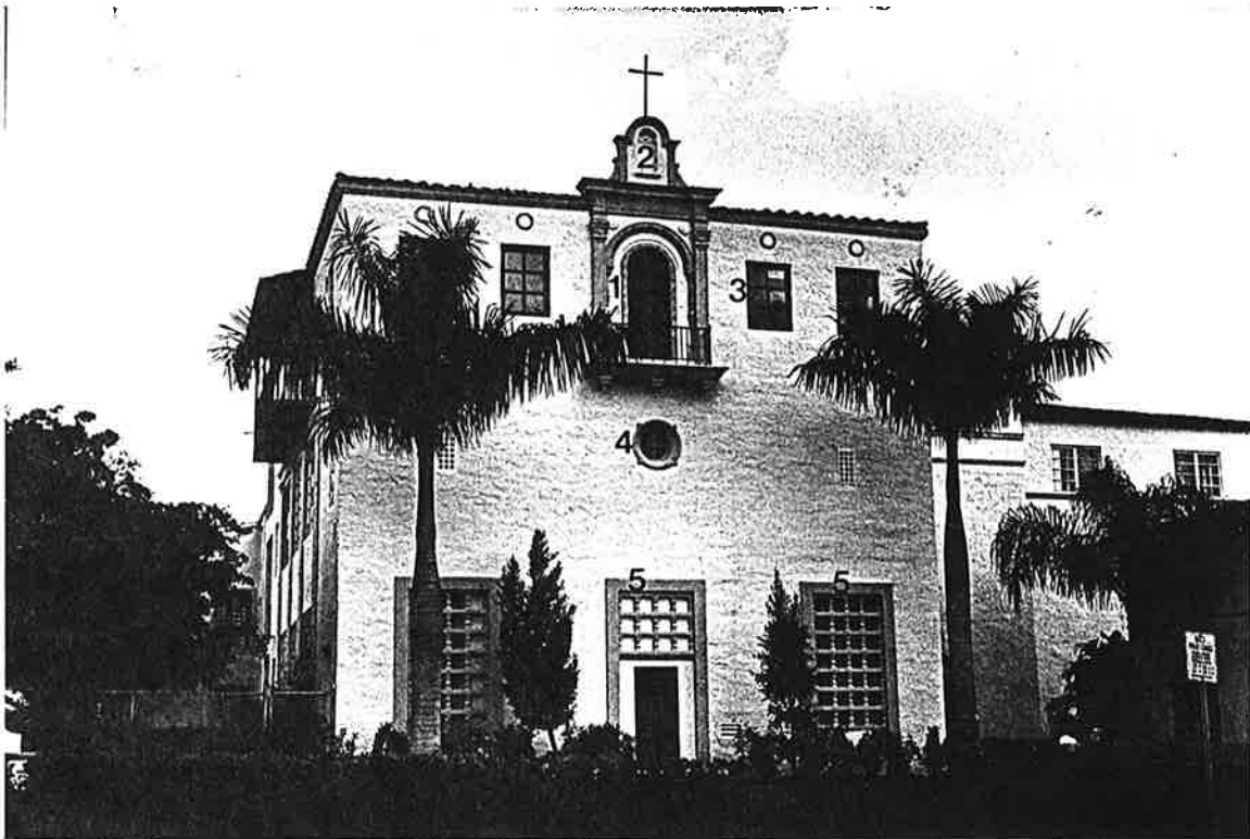
Original 1925 school, west elevation
