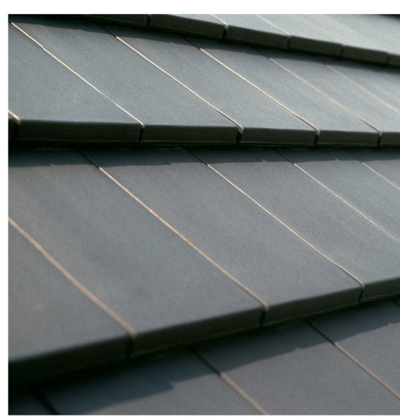
0705 FLAT ROOF CEMENT TILE
