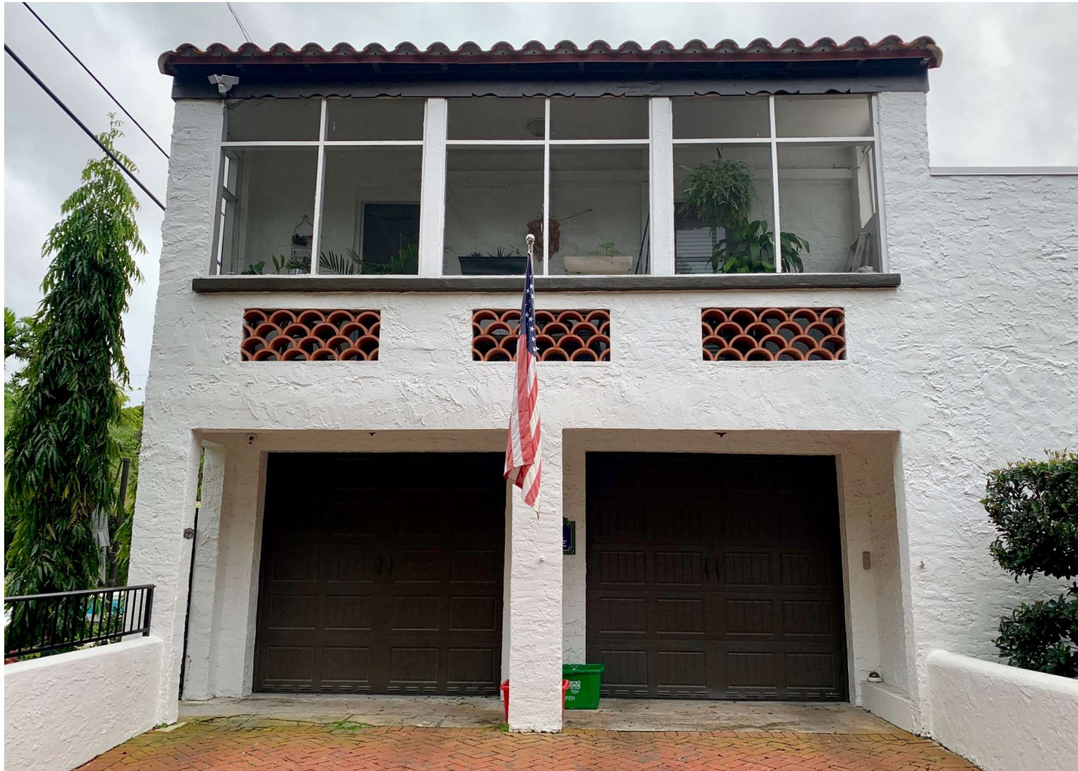
North Façade – After
