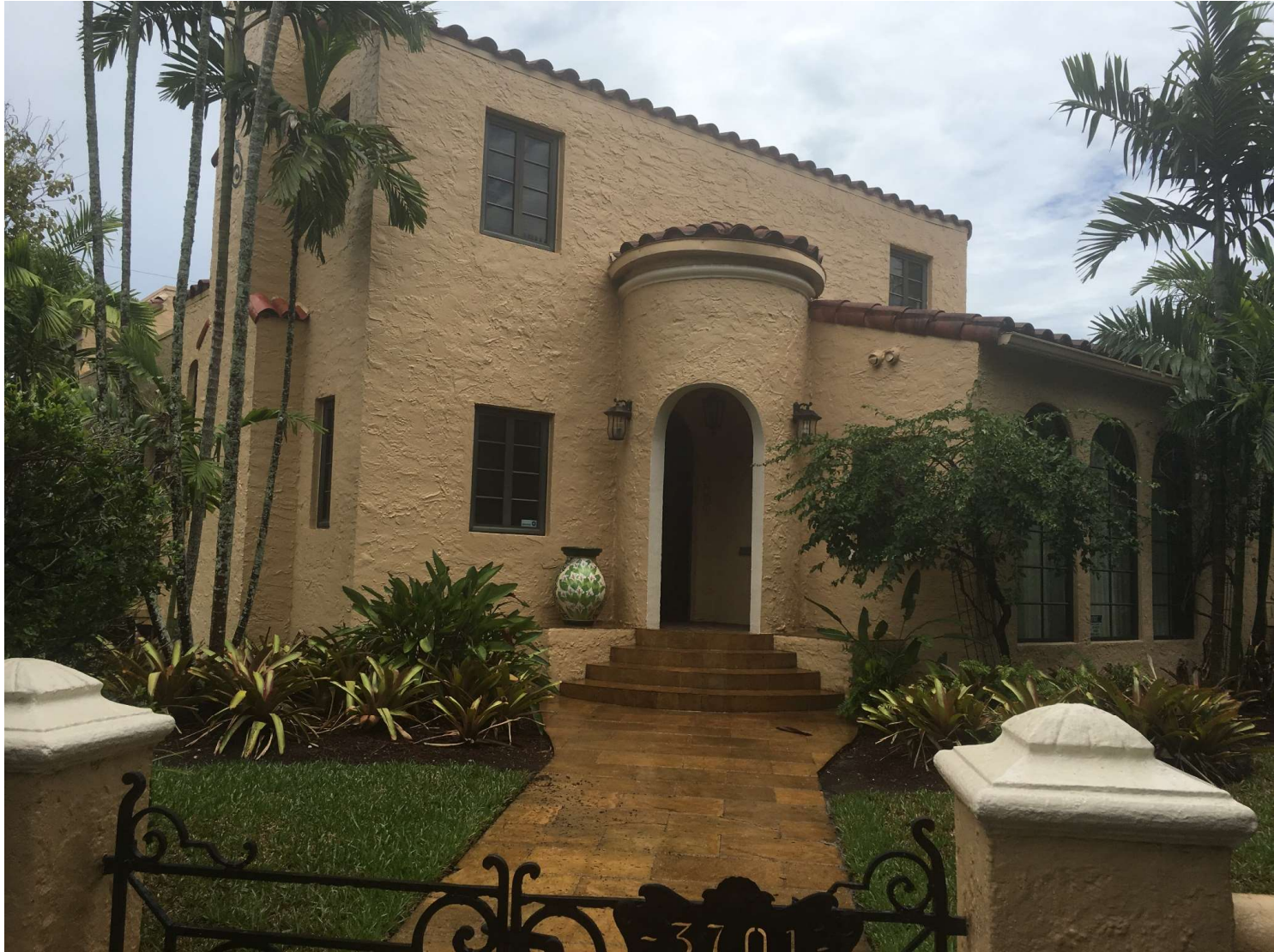
Northwest Corner Entry - Before
