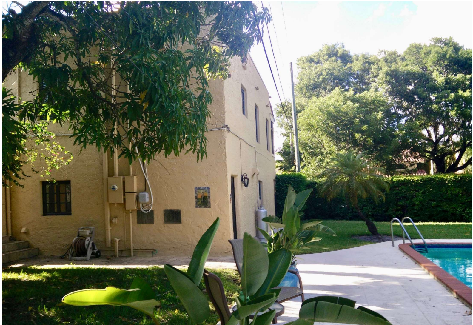
South Façade (Back of Garage) – Before
