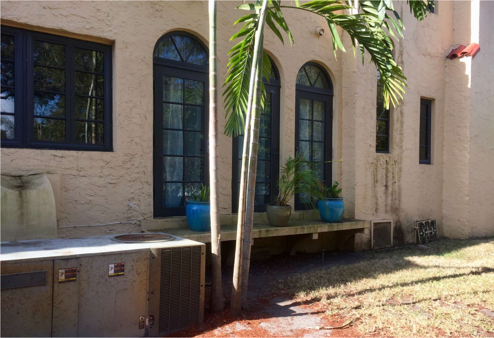
North Façade – Before
