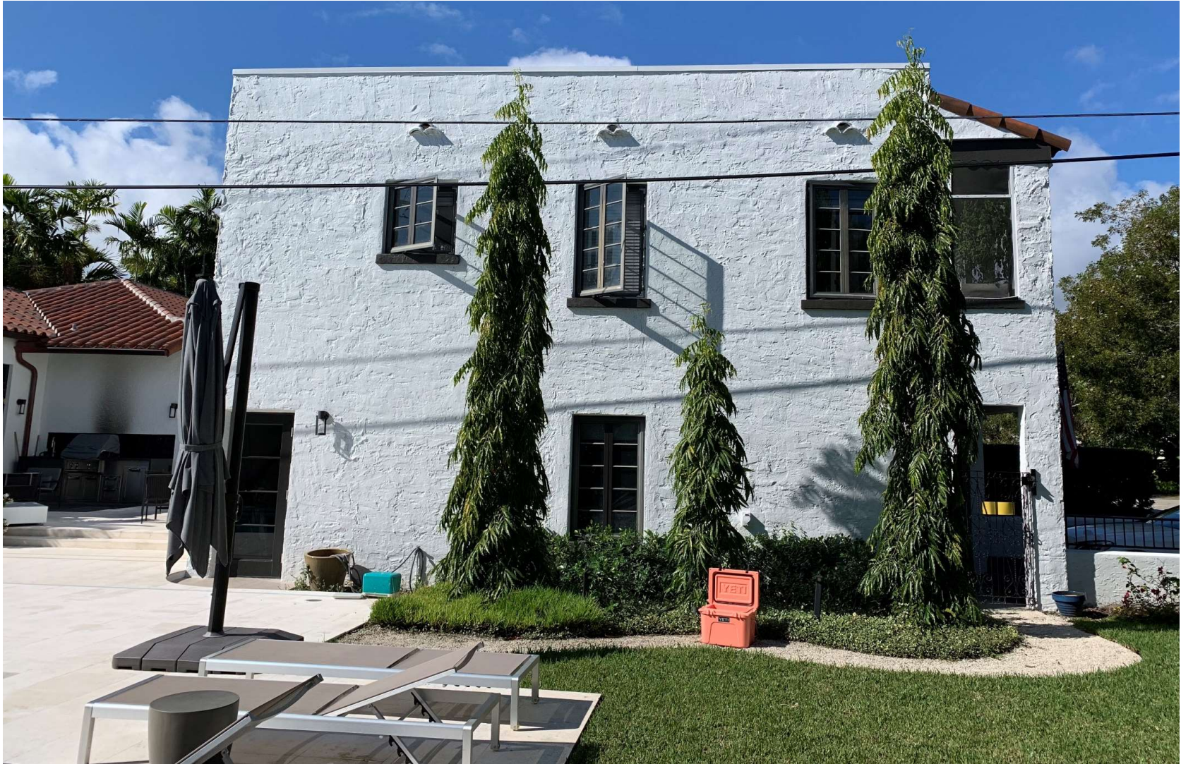
East Facade – After
