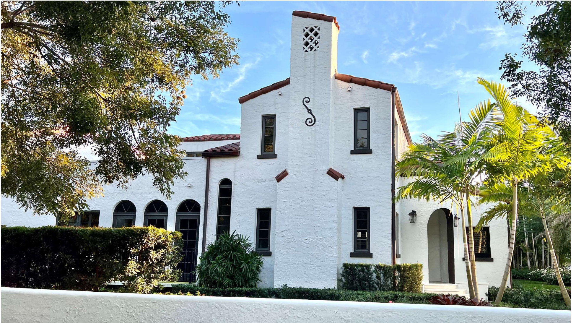
North Façade – After
