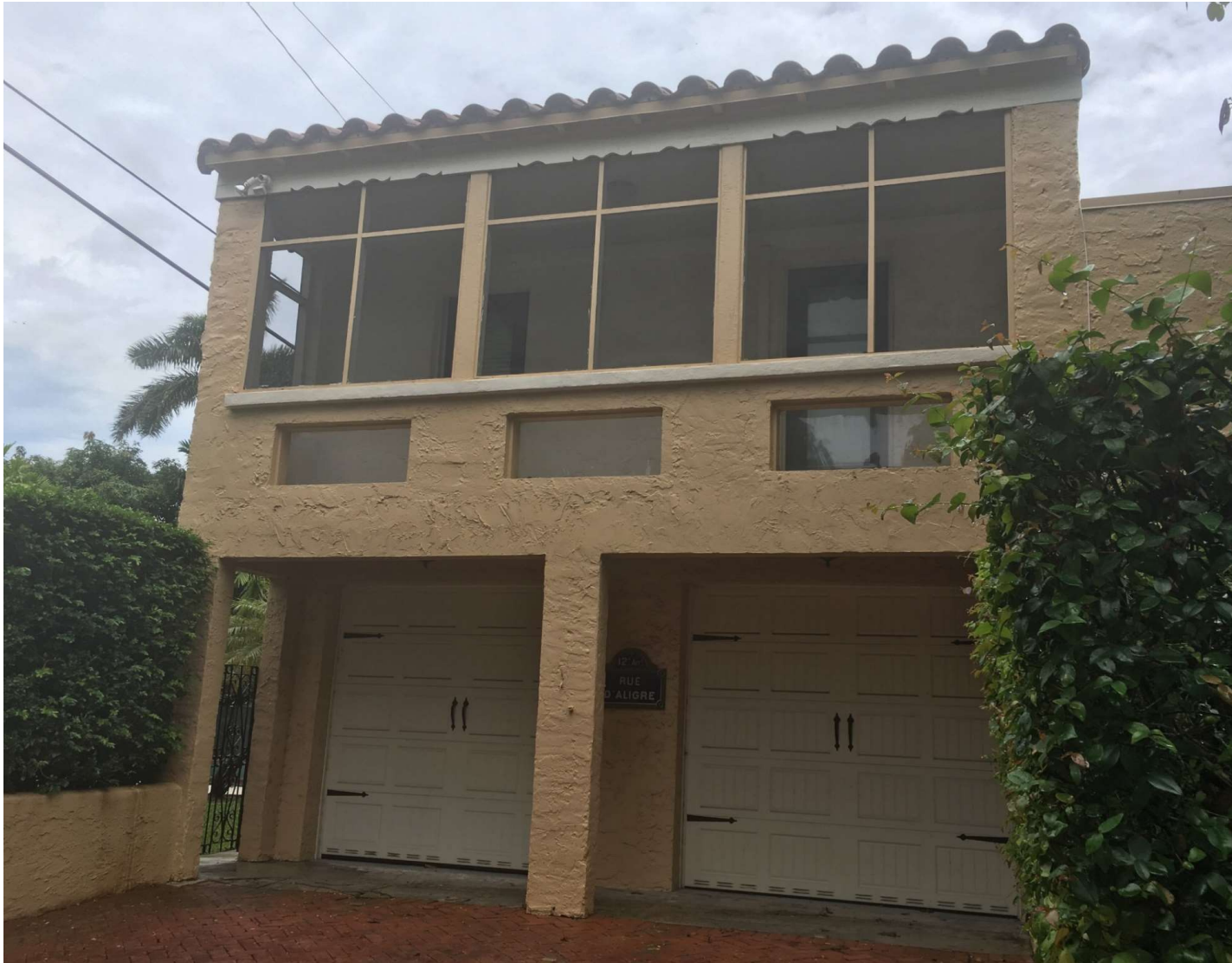
North Façade – Before
