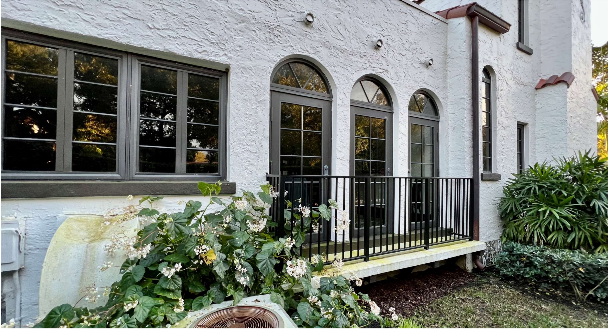
North Façade – After
