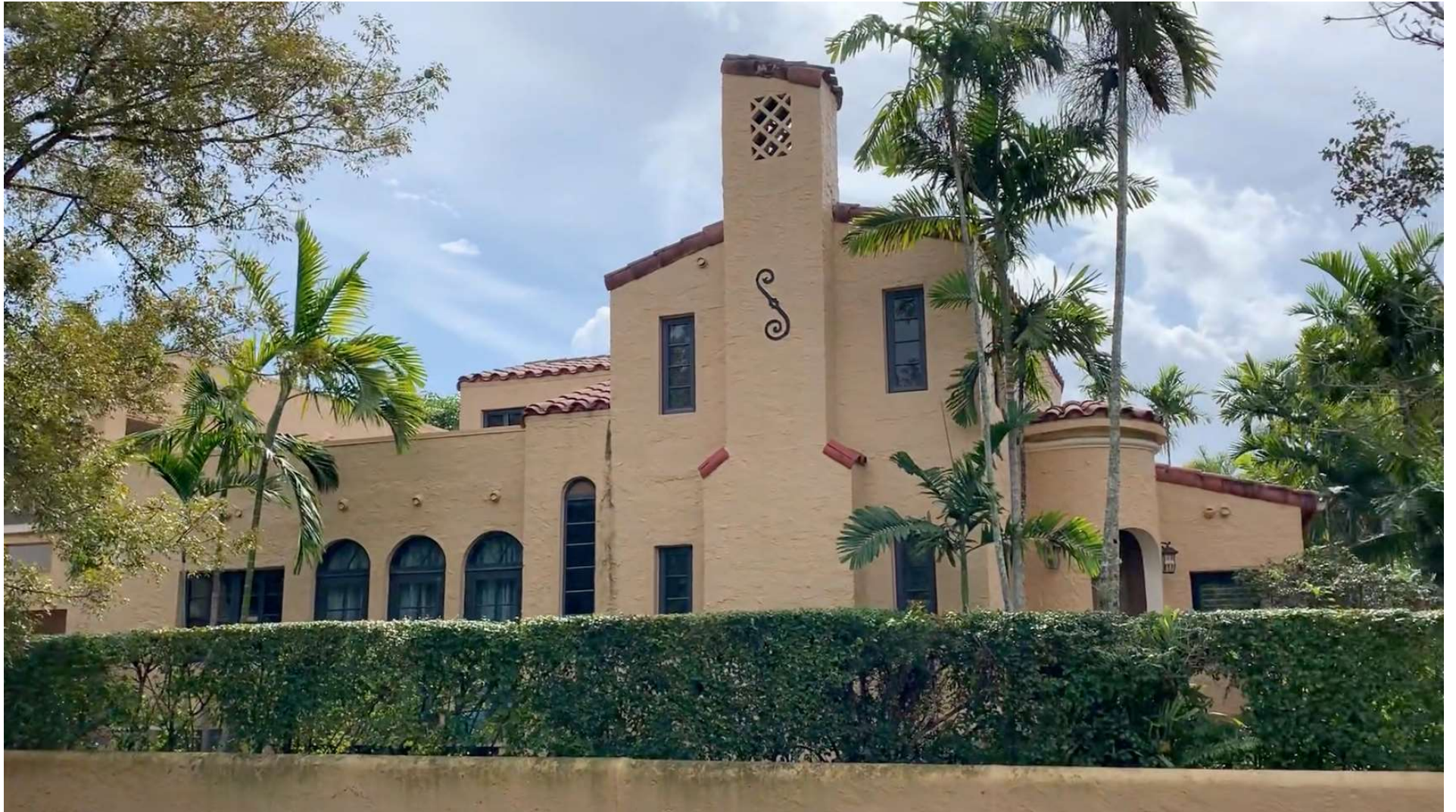
North Façade – Before
