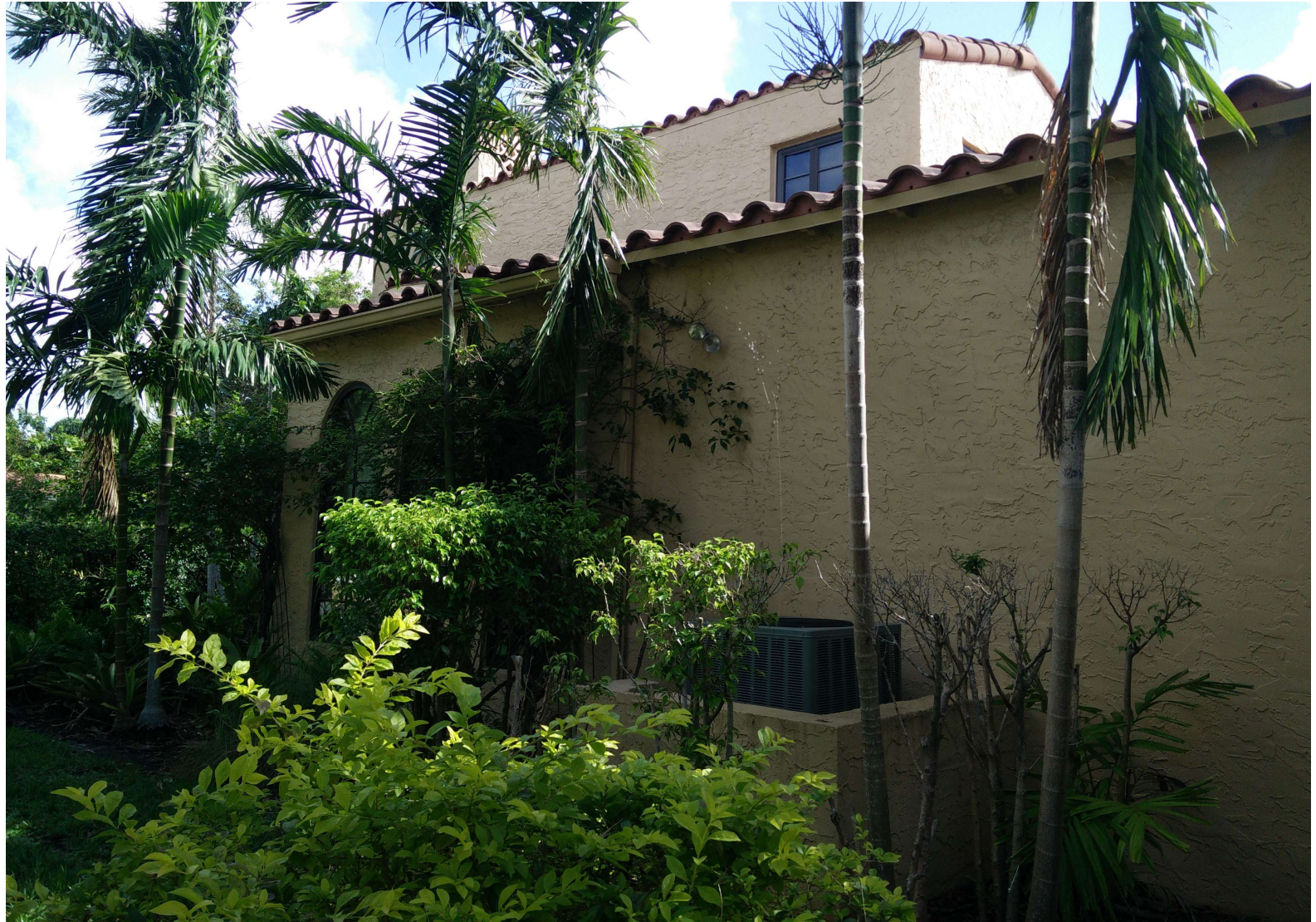
West Façade – Before
