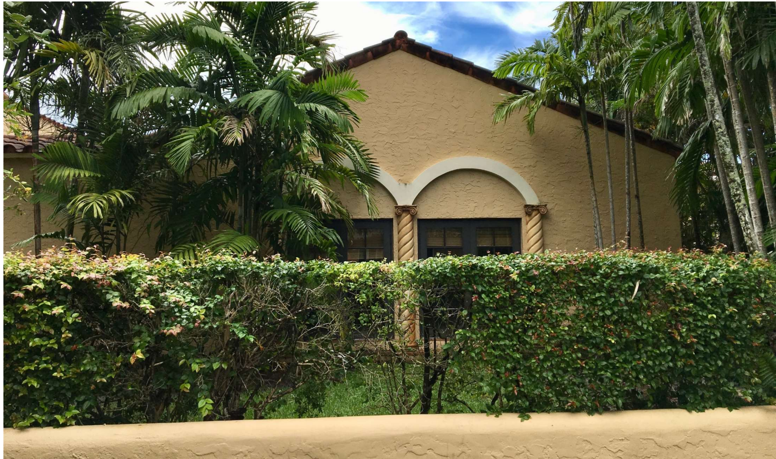
West Façade – Before
