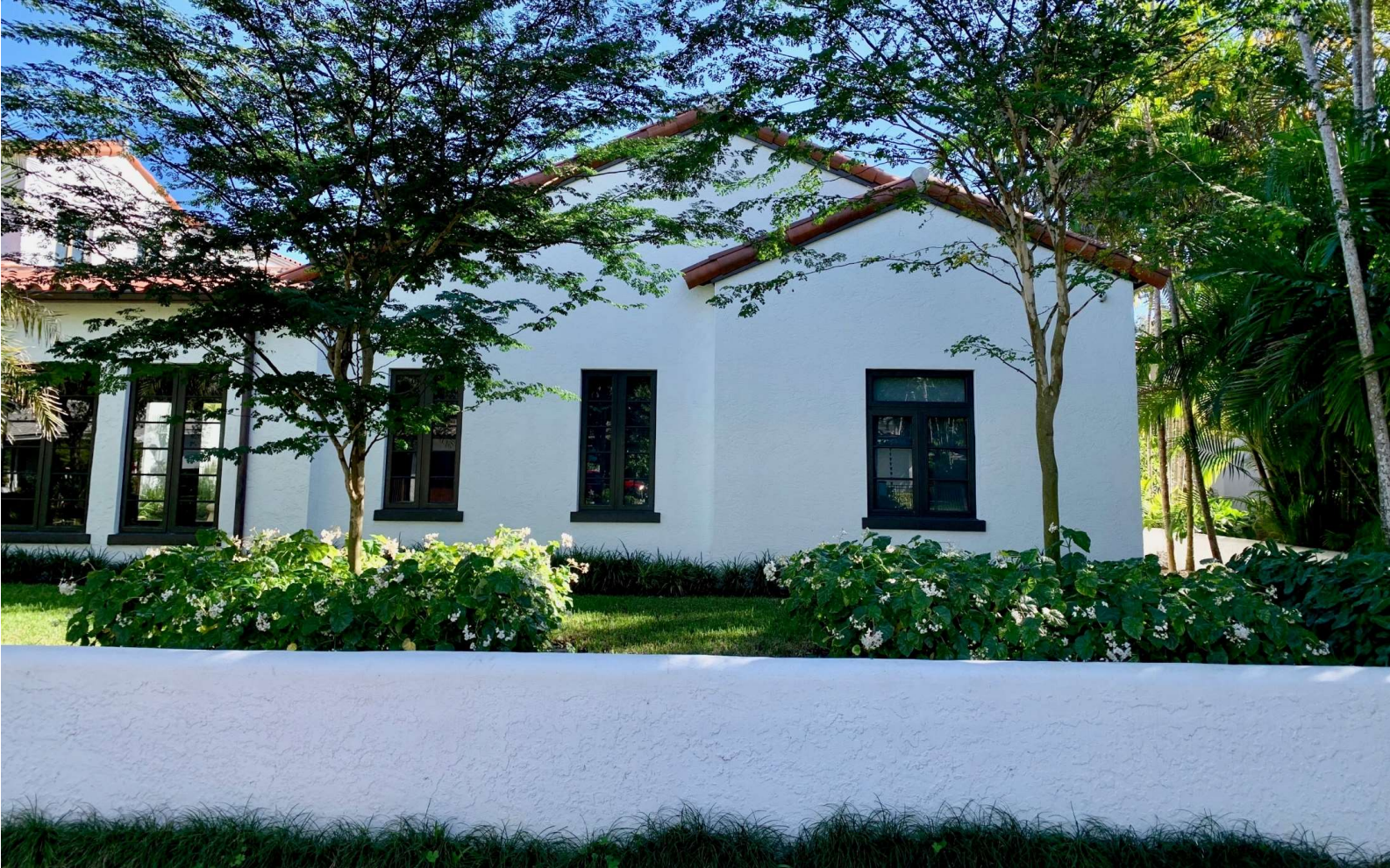
West Façade – After
