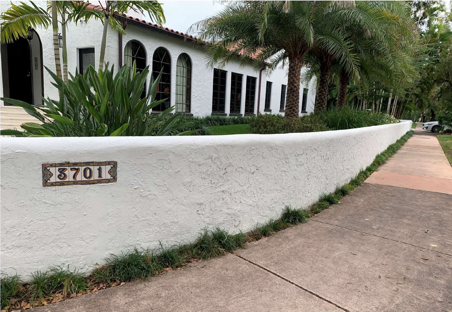
Northwest Corner and Perimeter Wall – After
