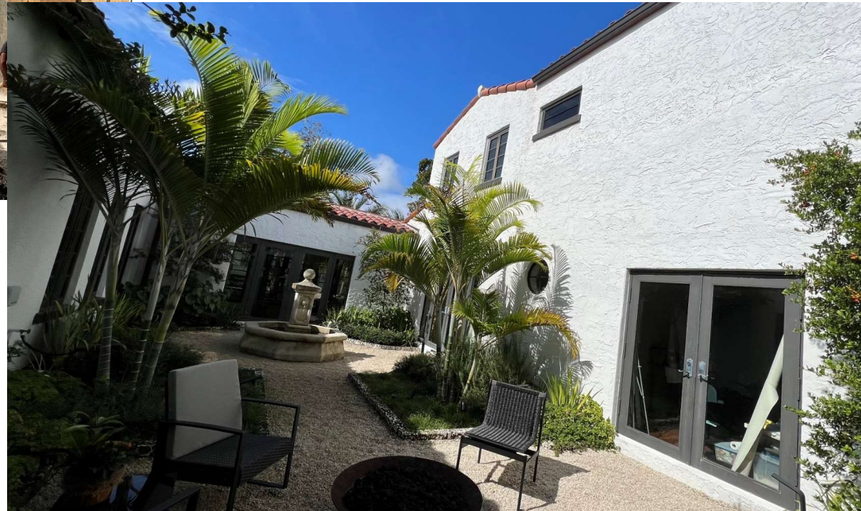
South Façade – Before and After
