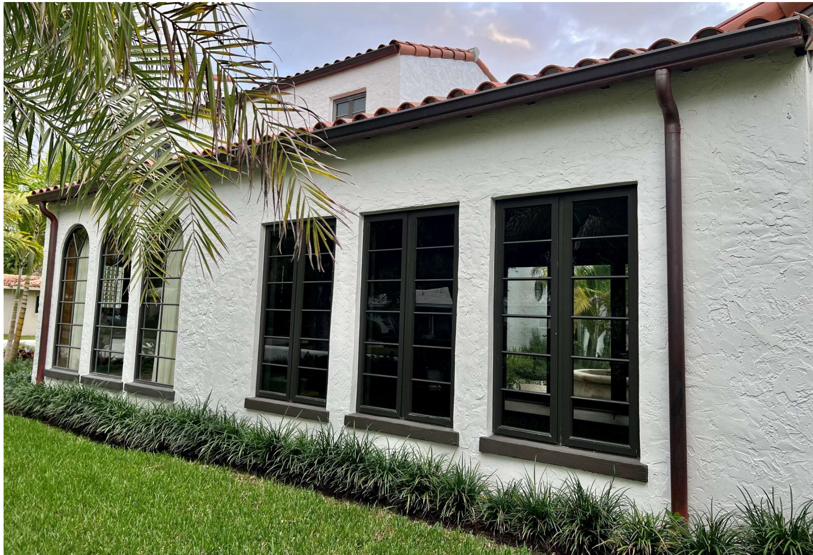
West Façade – After
