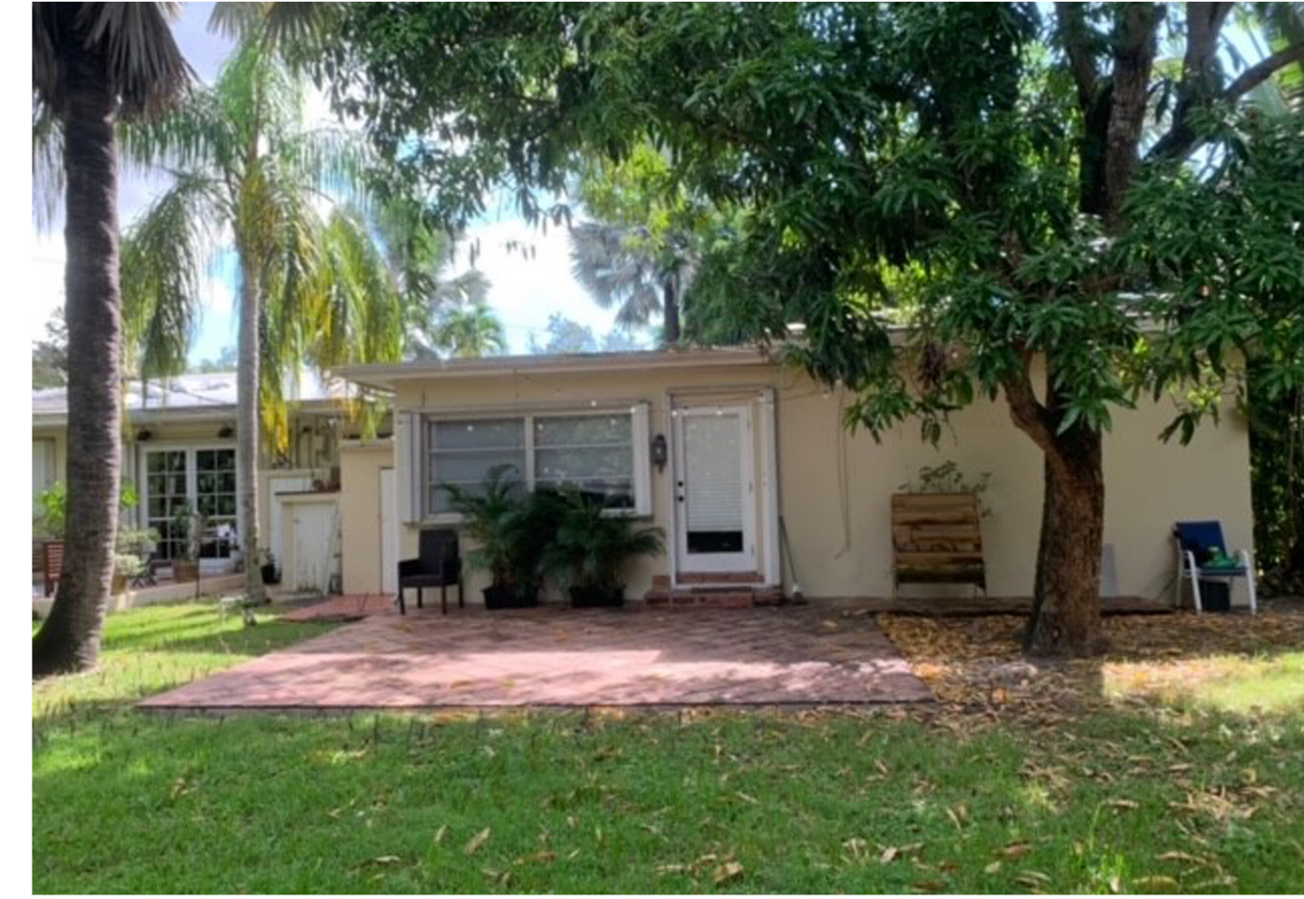
3520 Segovia Street - Rear/West
