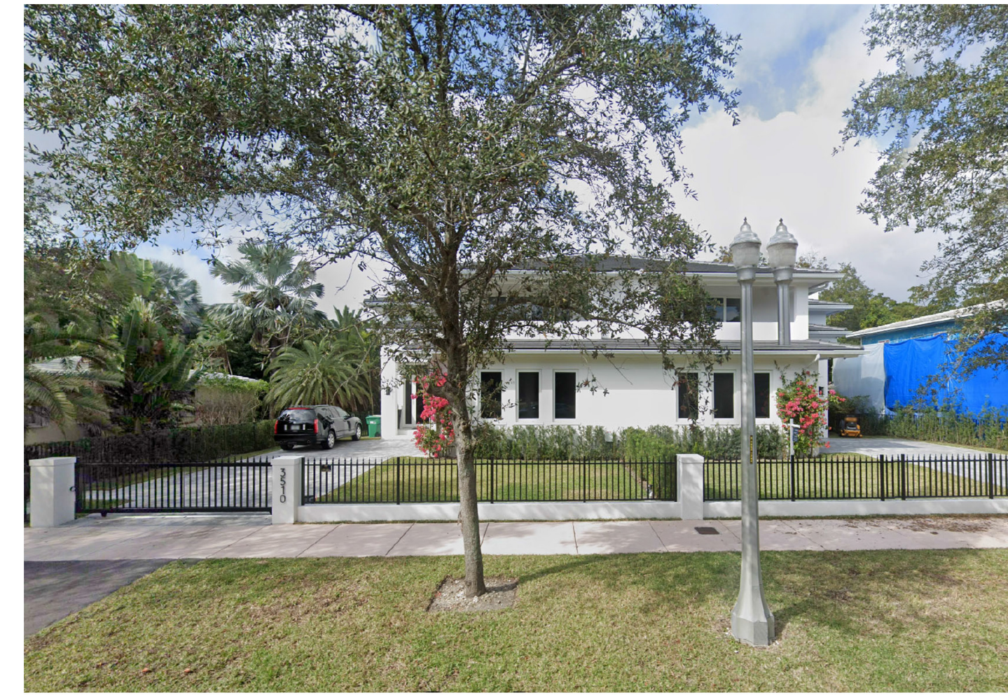
Adjacent Property - 3508 Segovia Street - Front
