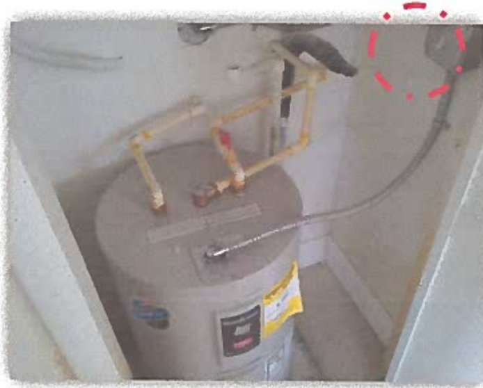
Add a means of disconnect (switch) to water heater or air handler.
