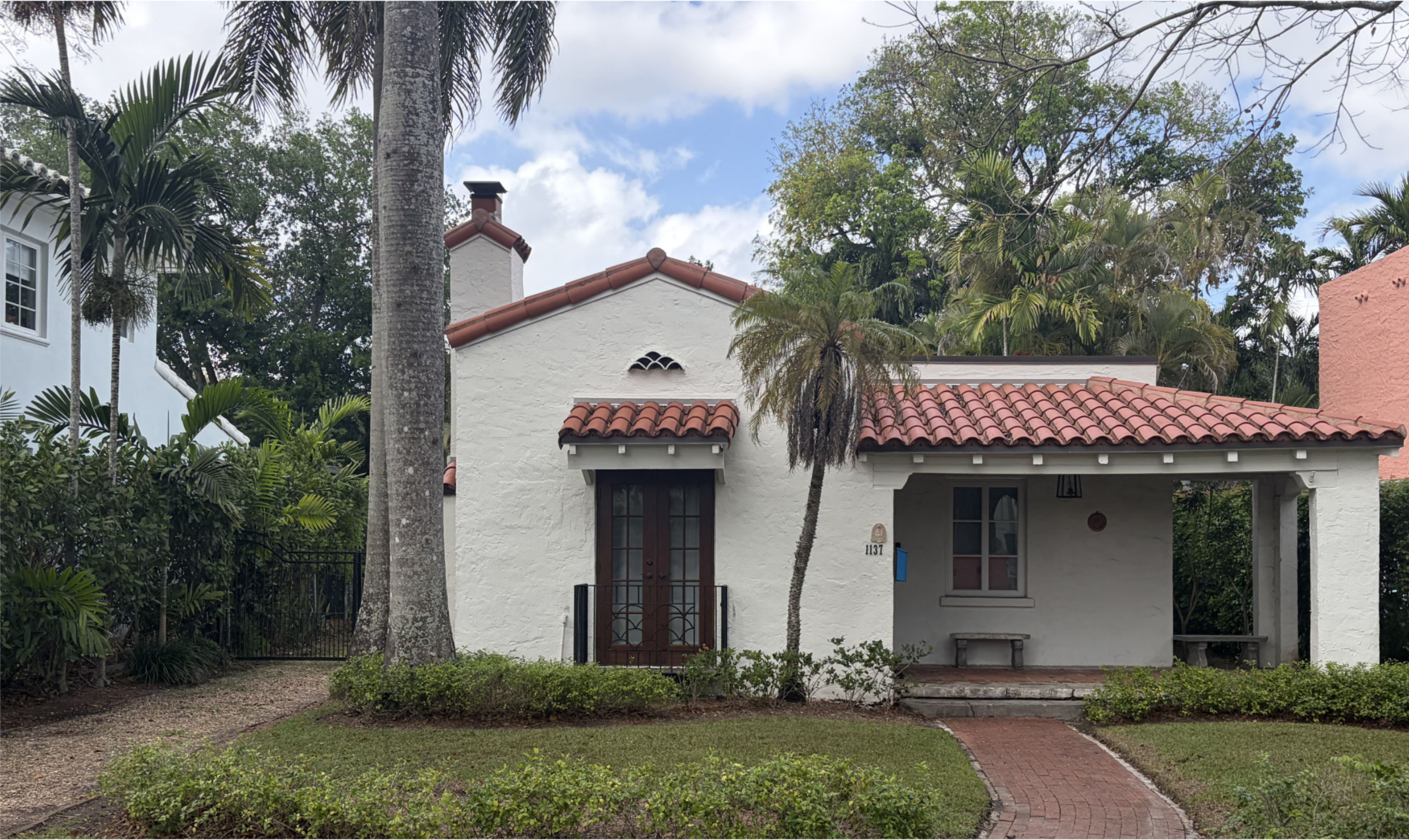
Existing front elevation from street
