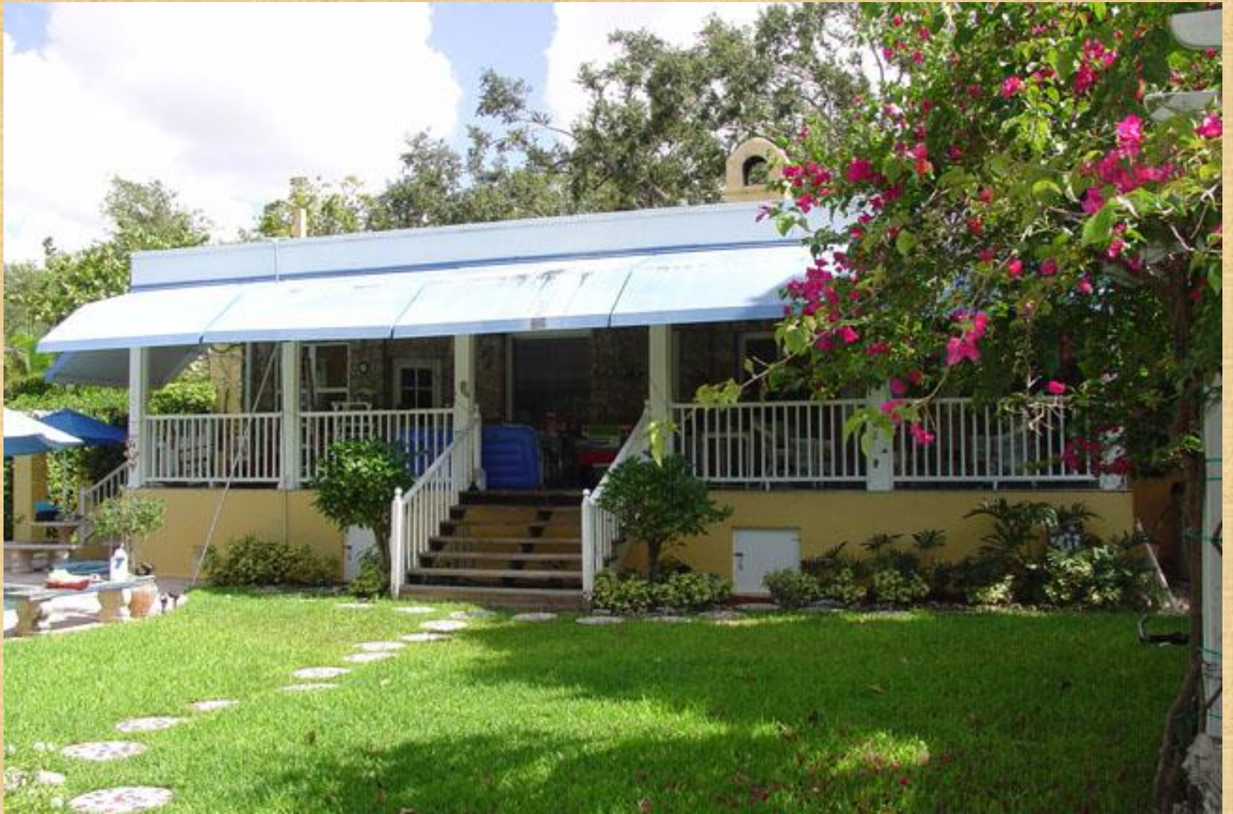
South Façade - Before
