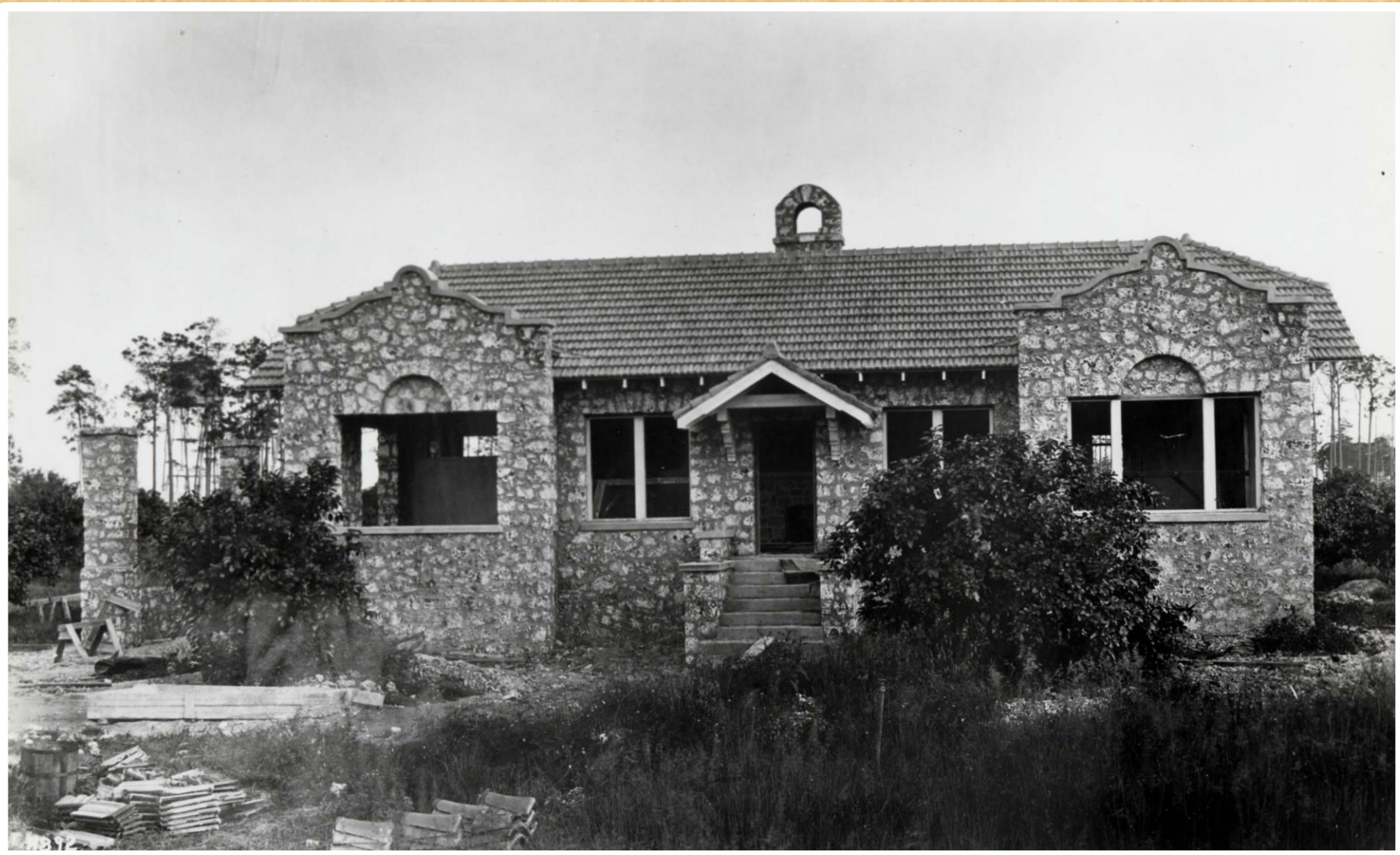
1254 Coral Way Under Construction
