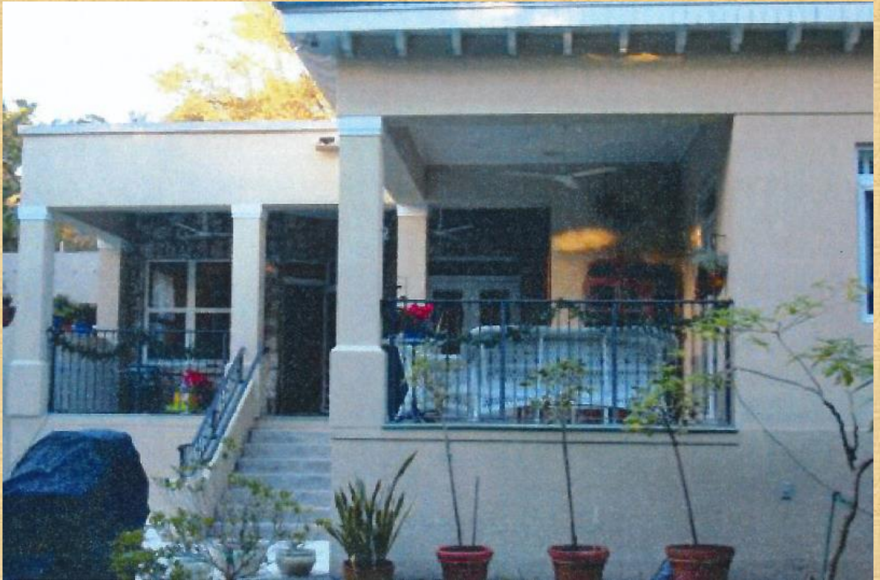
South Façade - After
