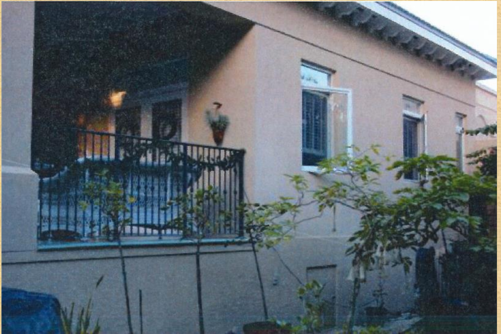
South Façade - After
