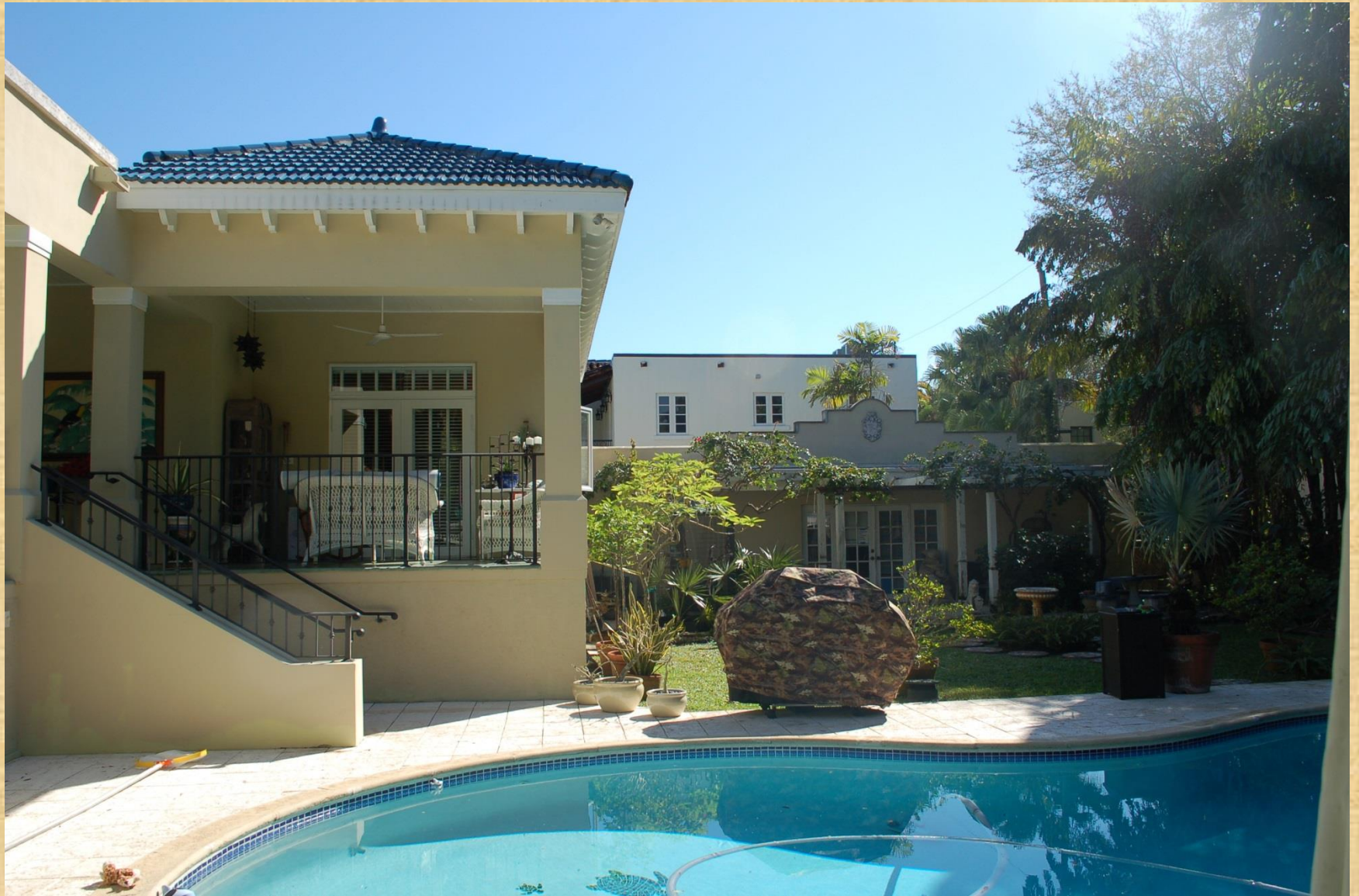
West Façade - After
