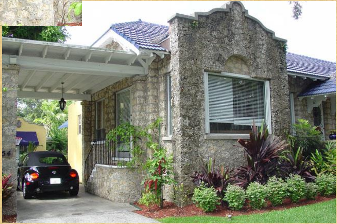
Carport Area - Before
