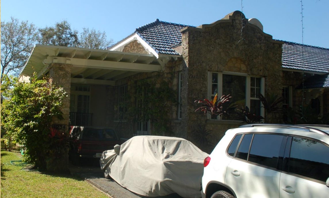
North Façade - Carport
