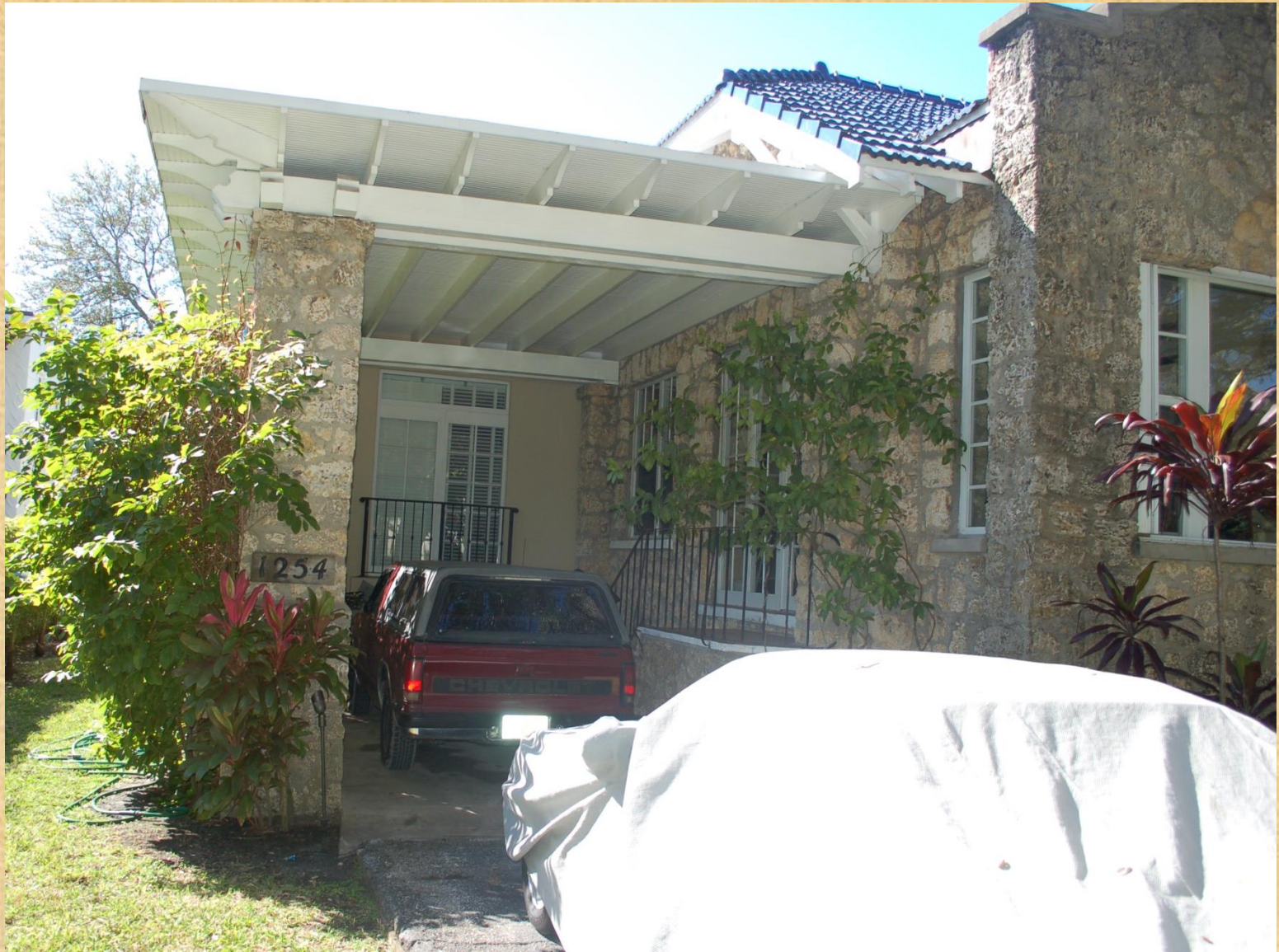
Carport Area - After
