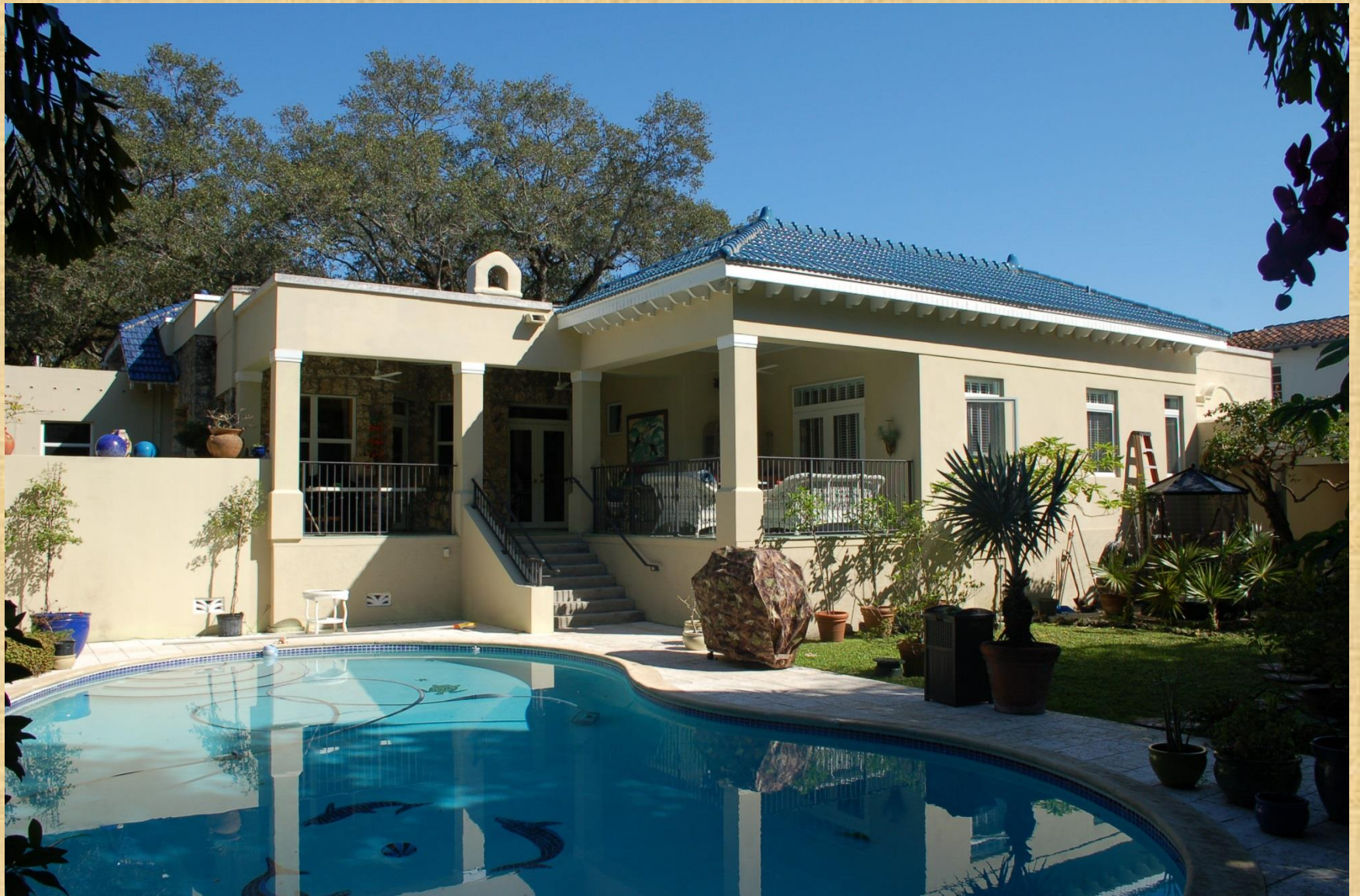
South Façade - After
