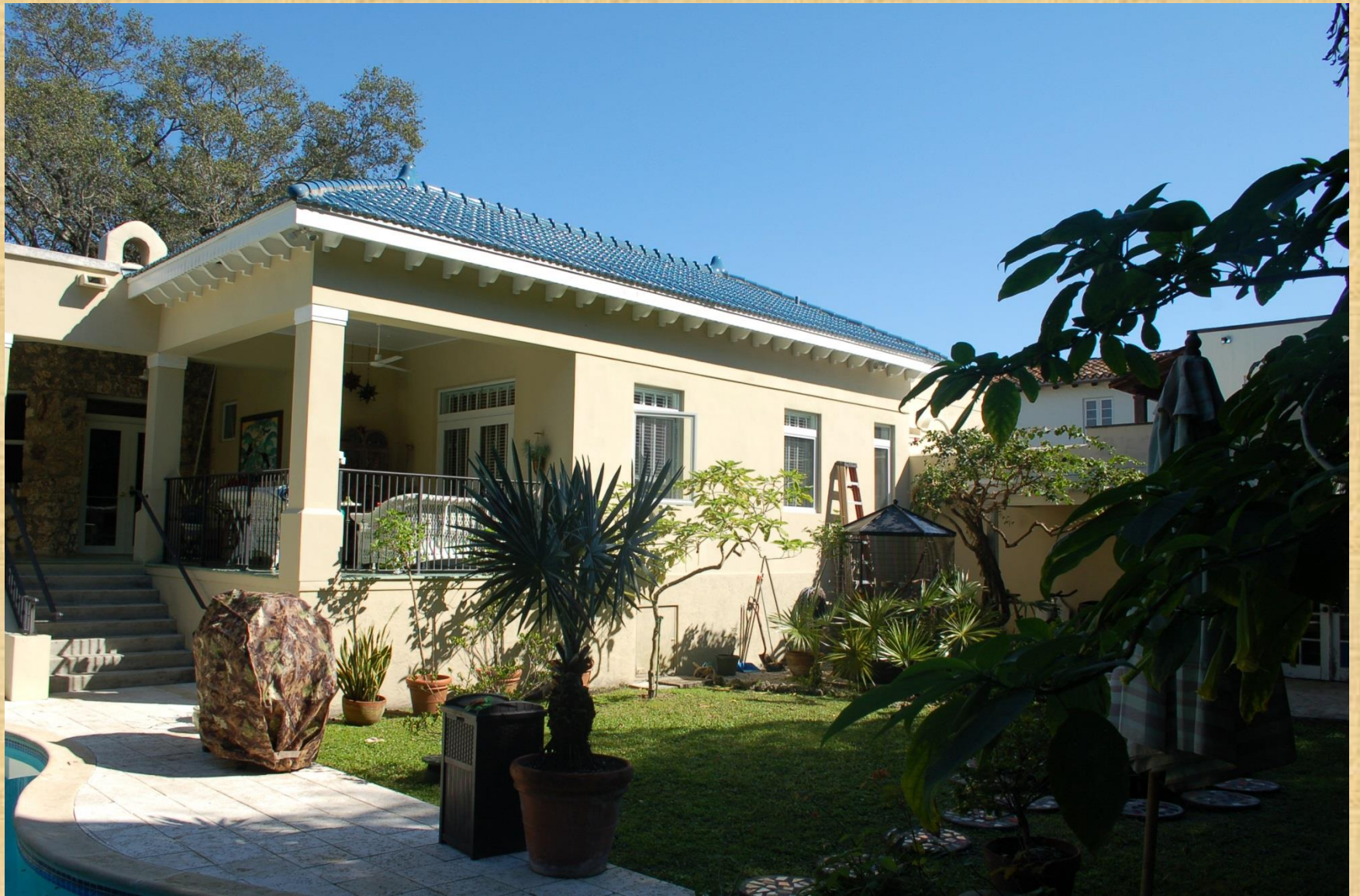
South Façade - After
