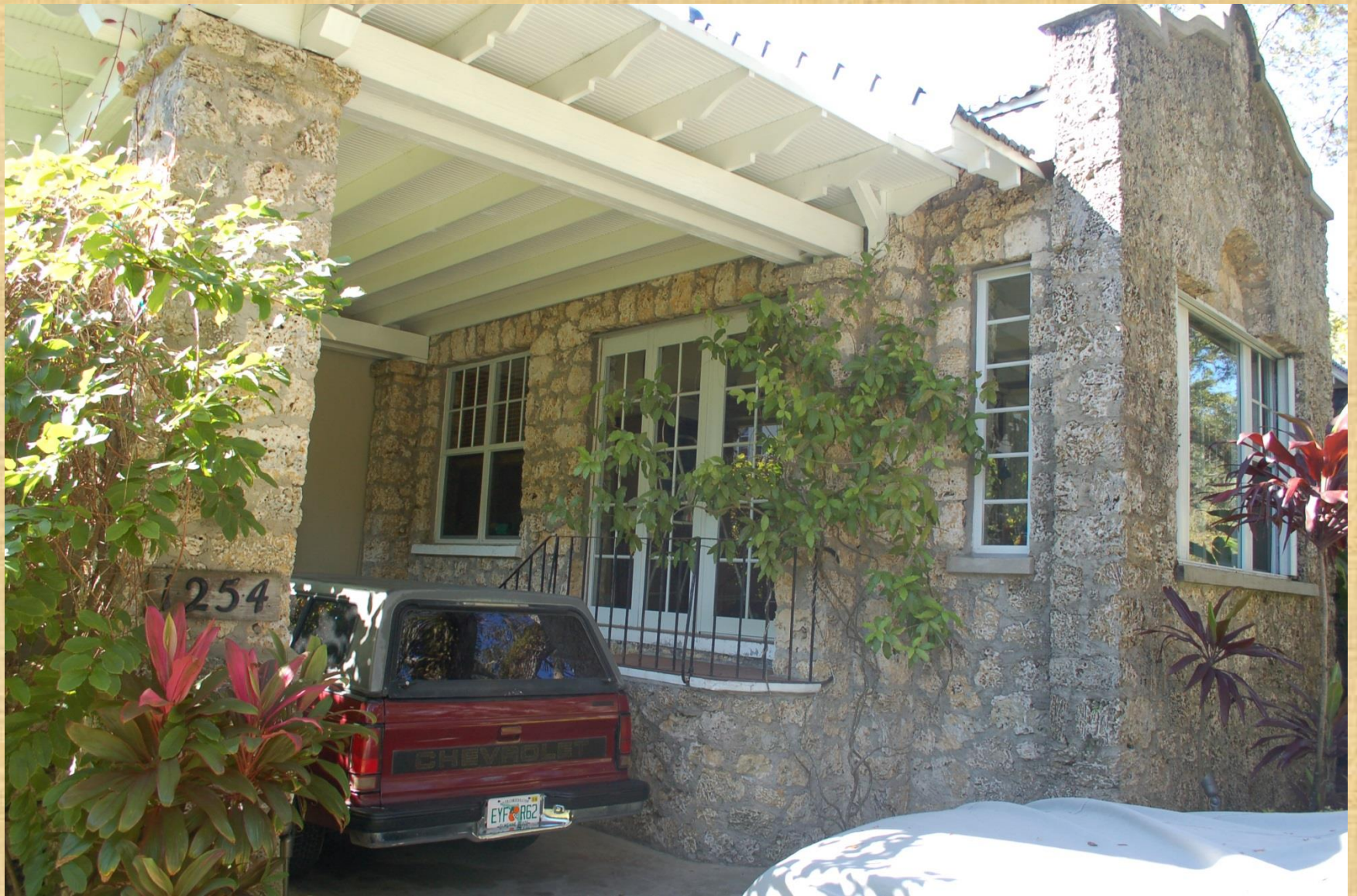
Carport Area - After
