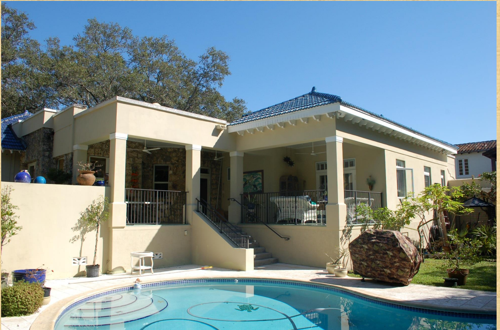
South Façade - After
