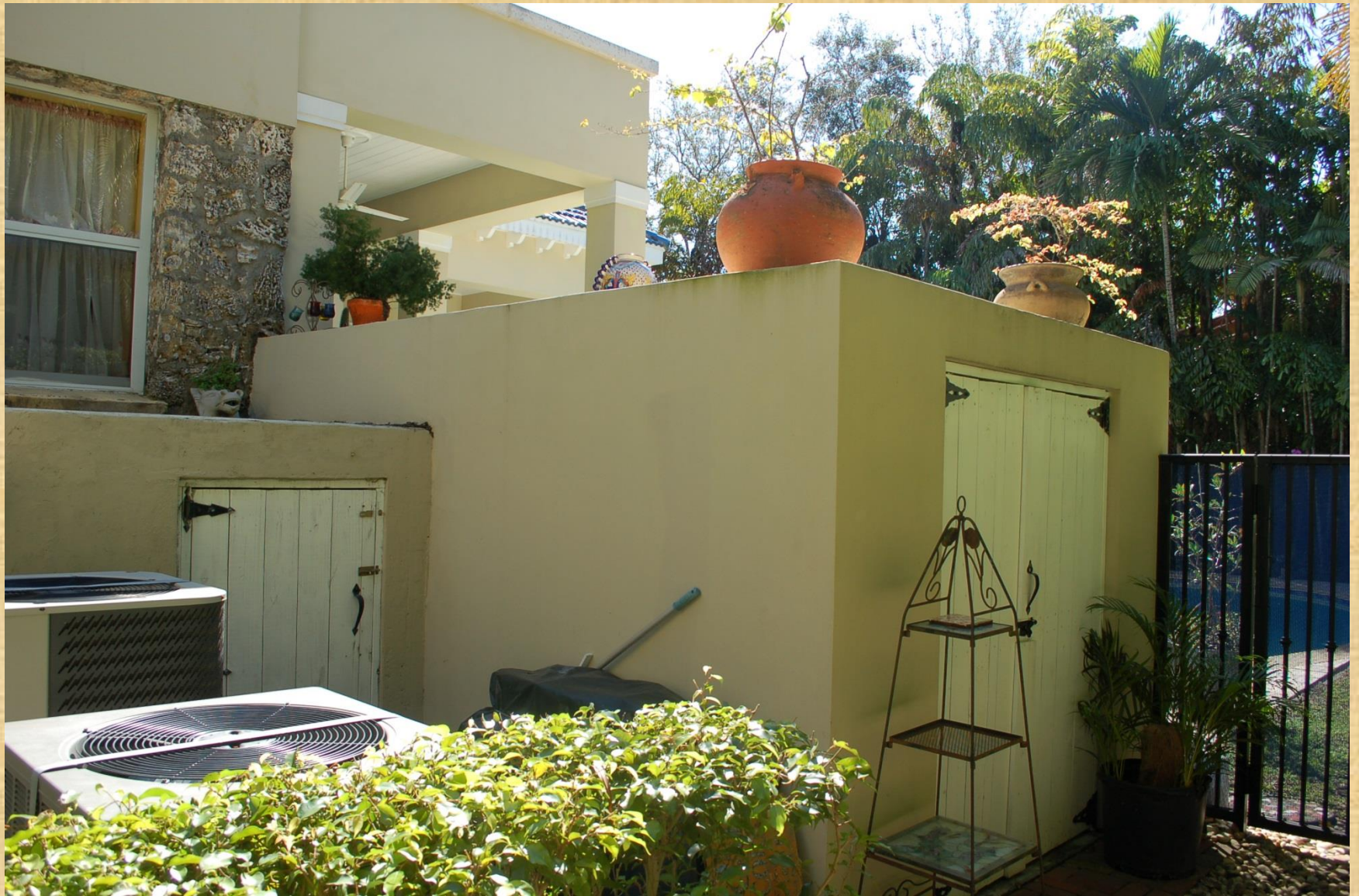
West Façade - After
