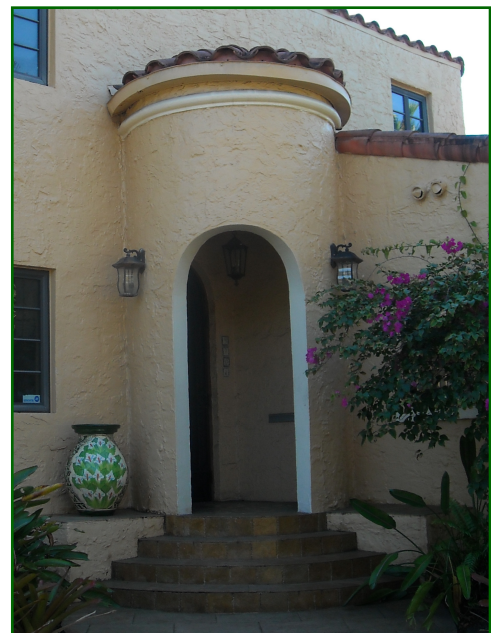
Figure 8: Front Entry Tower, 2018
