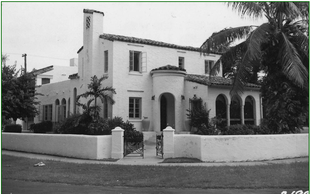
Figure 1: 3701 Durango Street, Front Facades, looking southeast, c. 1940
