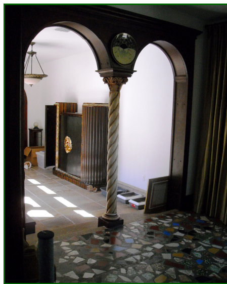
Figures 21: Twisted Columns, Enclosed Porch, Front Façade Top: Permit #1749 Drawing, 1925 [left]; Current Condition, Exterior, 2018 [right] Bottom: Current Condition, Interior, 2018: looking west [left]; looking south [left] Note: Original porch random tile flooring; same flooring as entry tower
