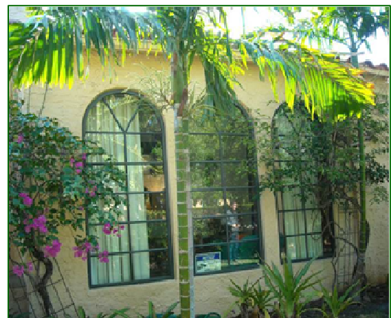
Figures 11: West Façade, 2018 Front entry tower and original door [top] Entry tower and north wall of projecting porch bay Note extant sill and decorative rafter tails below gutter [center] Porch bay, west wall, arched openings now enclosed [bottom]
