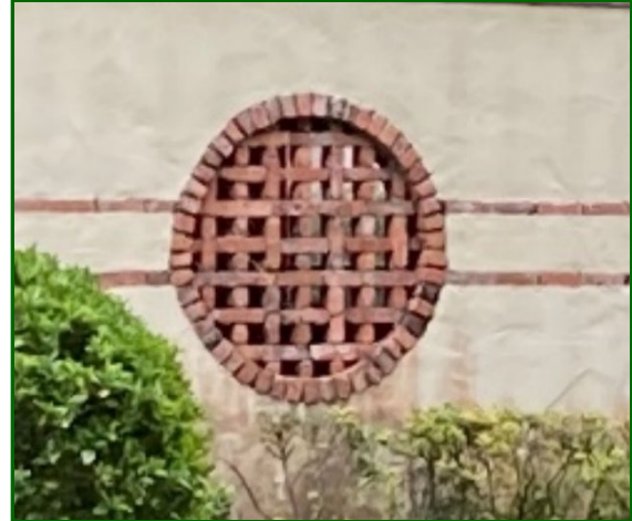
Figure 9: Garage ‘Porthole’ Brick Screen, 2024
