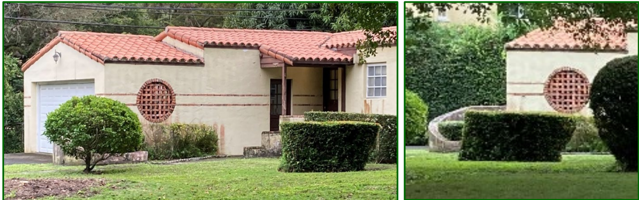
Figures 18: Northern Wing Containing the Garage, 2024
