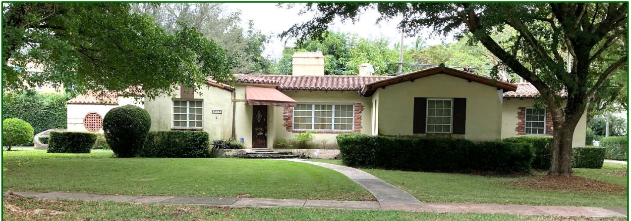
Figures 8: 3519 Toledo Street, Front (West) Façade c.1942 [top]; Current, 2024 [bottom]
