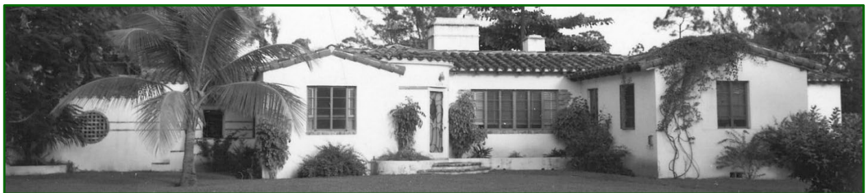
Figure 13: Front (West) Façade, c.1942
