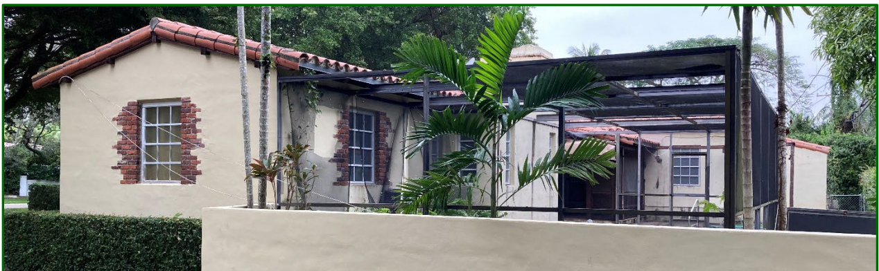
Figures 15: 3519 Toledo Street, 2024 From Top to Bottom: Front (West) Façade; From Southwest Corner of Property; Side (South) Façade; Rear (East) Façade From Escobar Avenue Looking North
