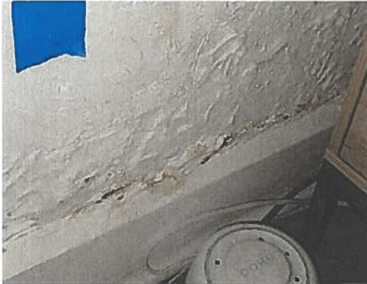
Moisture Stains Noted on Base Wall
