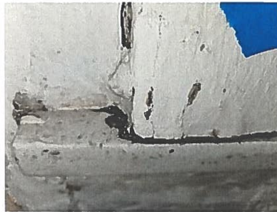
Damage And Mold Growth
