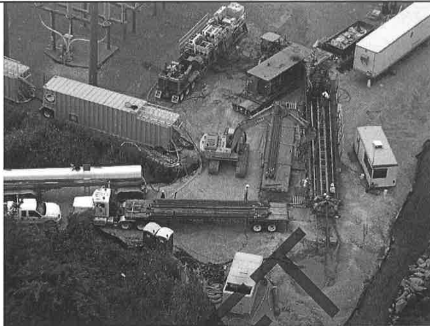
Figure 3-6 Typical HDD Setup
