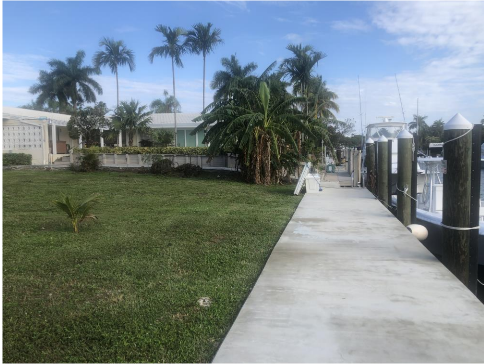
6935 SUNRISE COURT - REAR SEAWALL (NORTH )
