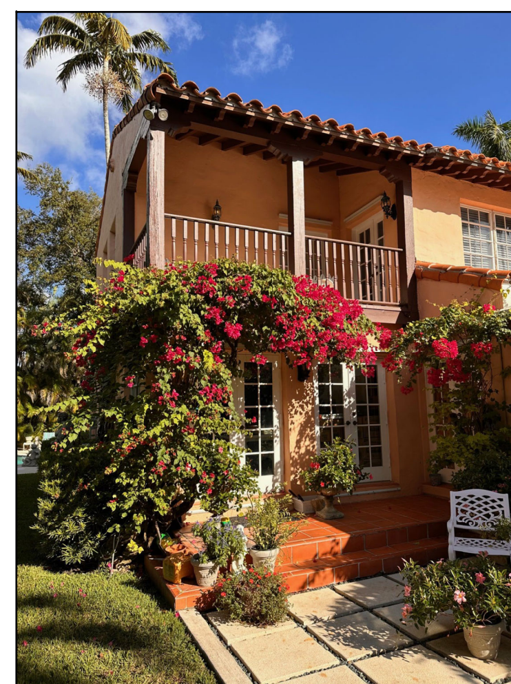
REAR PORCH DETAIL
