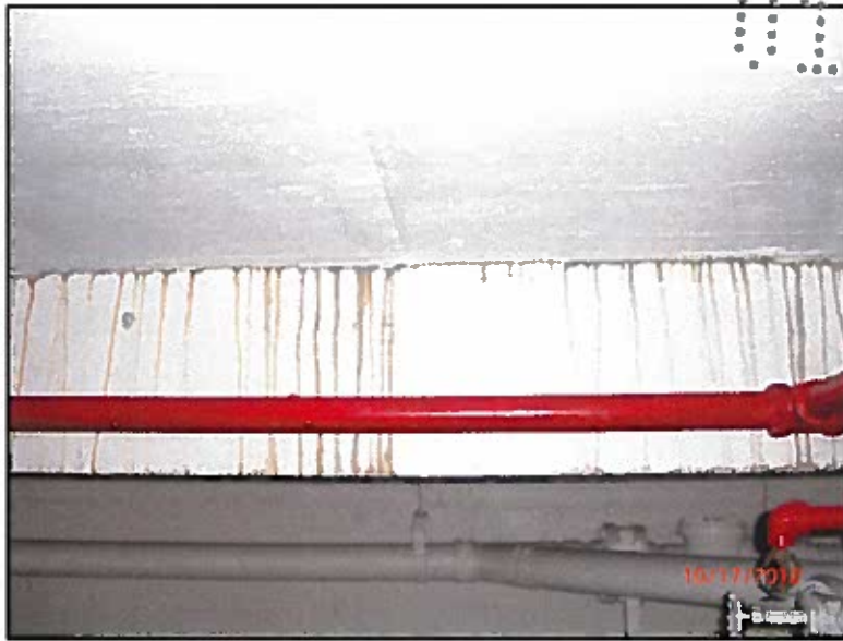
PHOTO # 25: trench drain drop ceiling between Parking Spaces 52 & 61
