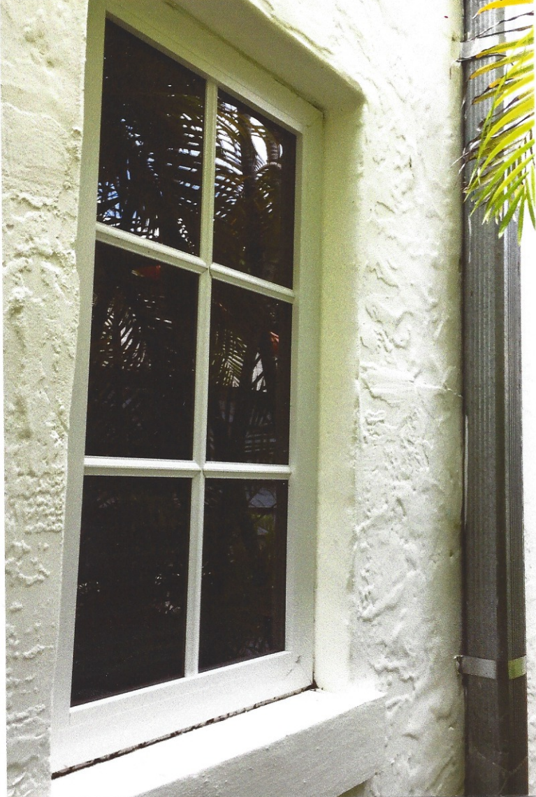
Feature: 7 Bathroom Window Elevation: East-side Photo: 9
