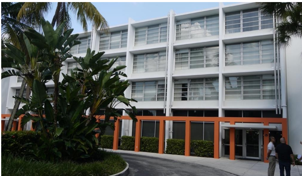
Fig. 7 (below): Eaton Hall, center wing east façade 2025. Note blank metal panels replacing original glass panes within awning windows on 2 nd 3 rd 4 th floors, non-historic window walls on the first floor, vertical metal bars of uncertain use, and the orange grid penetrating original awnings.
