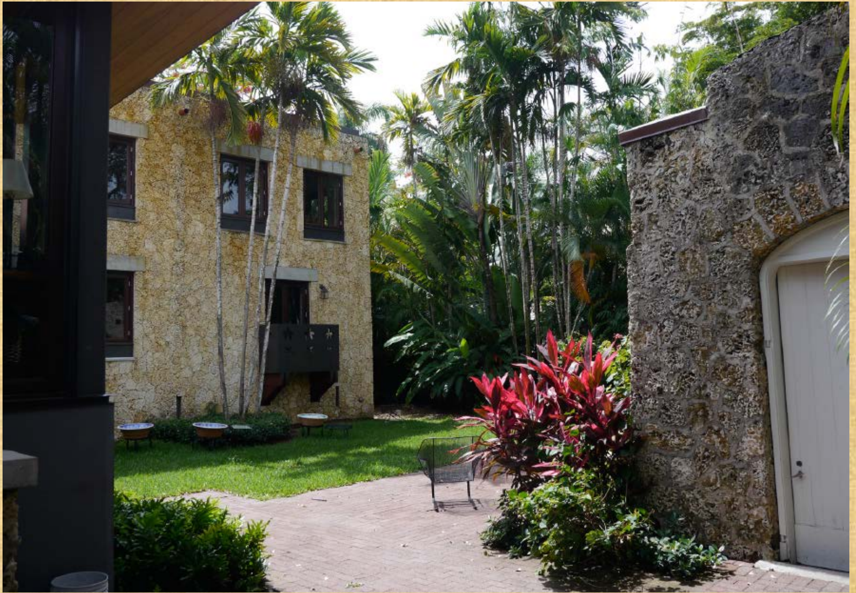
West Façade of Addition
