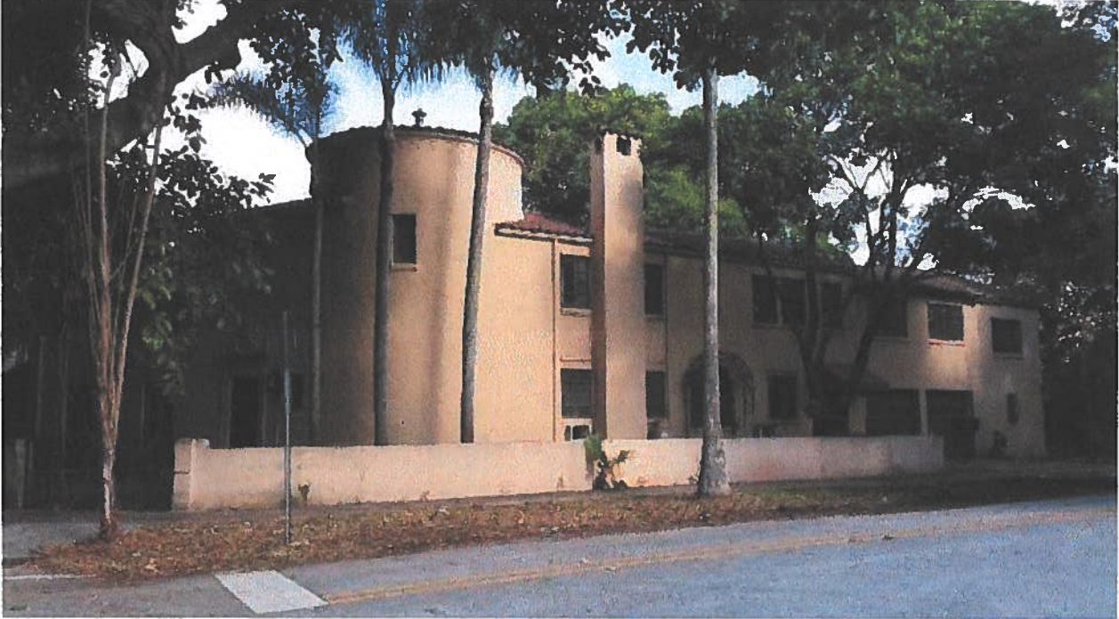
Elevation: East Existing Photo Number: 3
