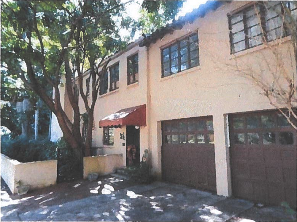
Elevation: East Existing Photo Number: 4
