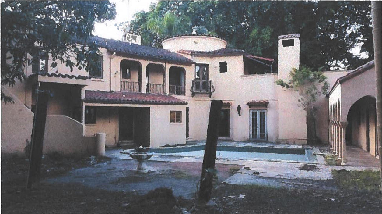
Elevation: North West Existing Photo Number: 7
