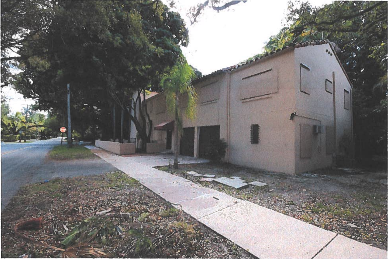
Elevation: East and North Existing Photo Number: 5
