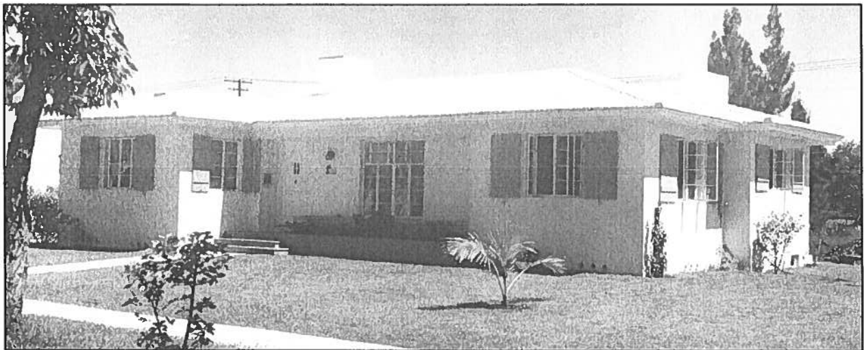
Figure 1: Photo ca. 1950s
