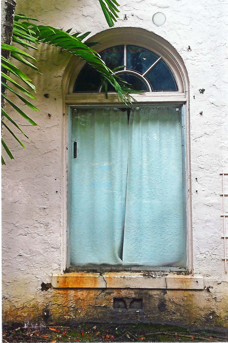
Feature 3 Arch Window Elevation: North-Front Photo: 3
