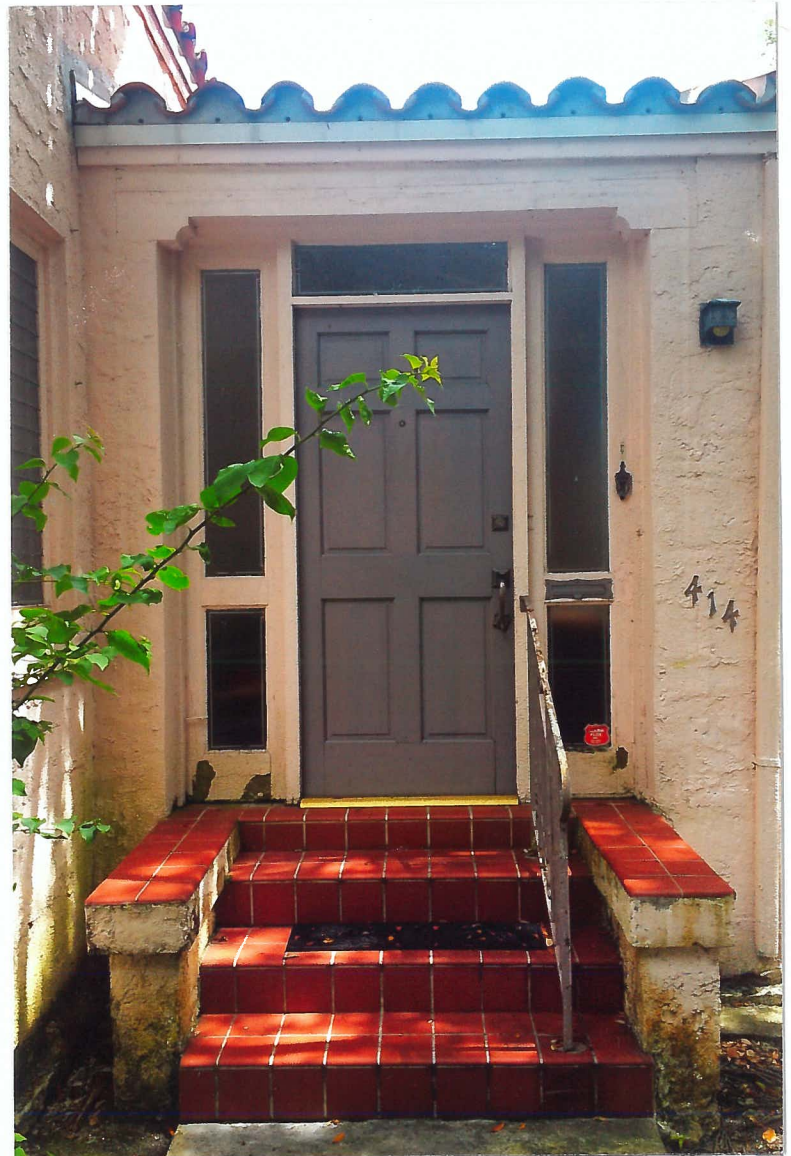
Feature: 2 Elevation: North Front Photo: 2
