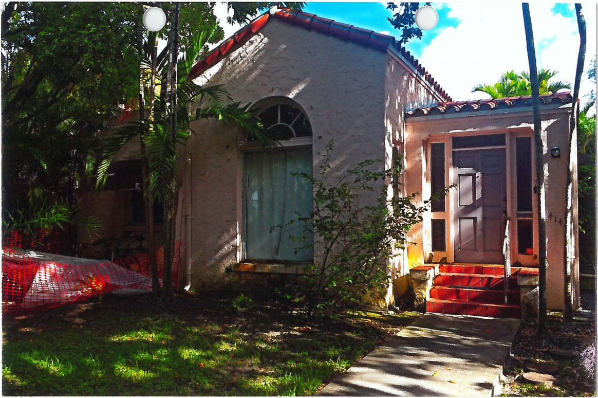
Feature: 1 Elevation: North Front Photo: 1
