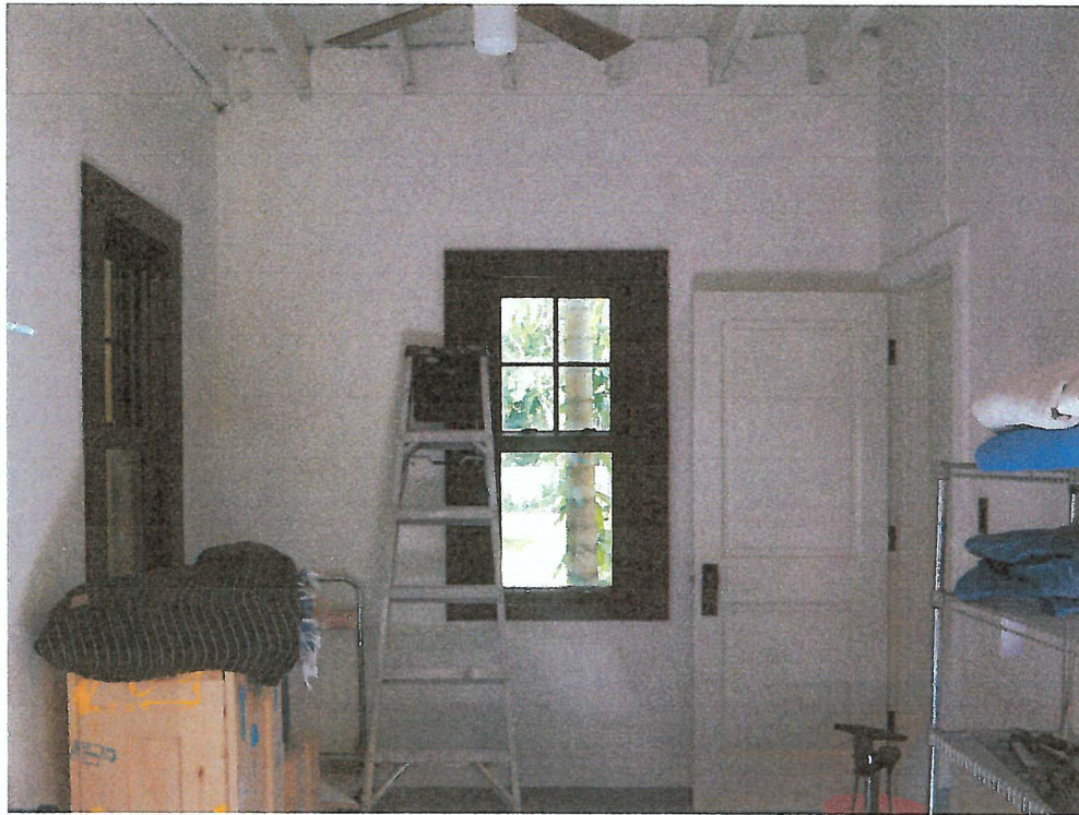
43. Room at Rear of Garage Looking Southwest
