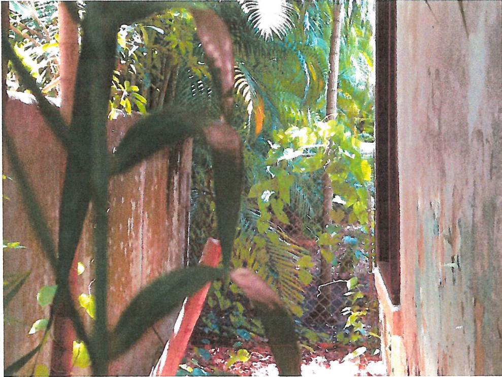
13. West Elevation of Existing Garage
