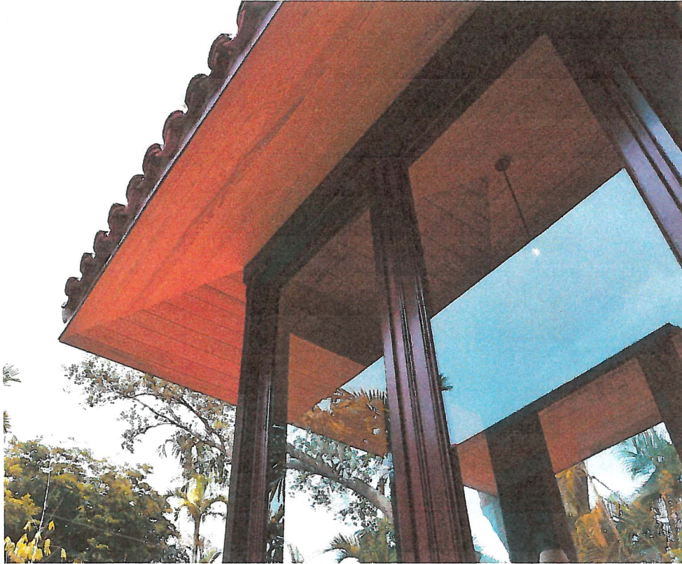
65. Window and ceiling details of glass kitchen nook
