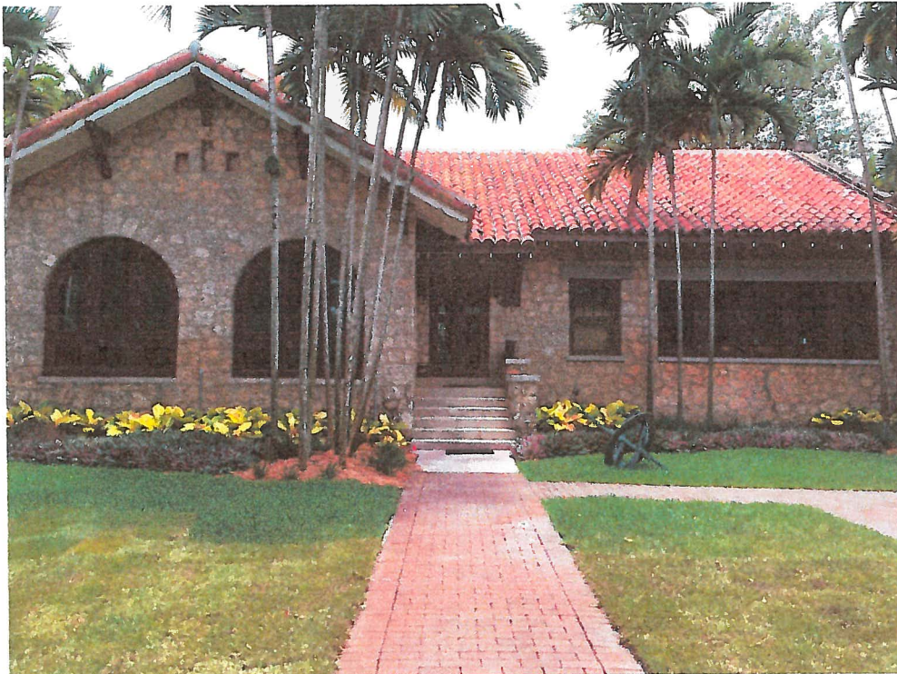
1. Front (North) Facade of Existing Residence
