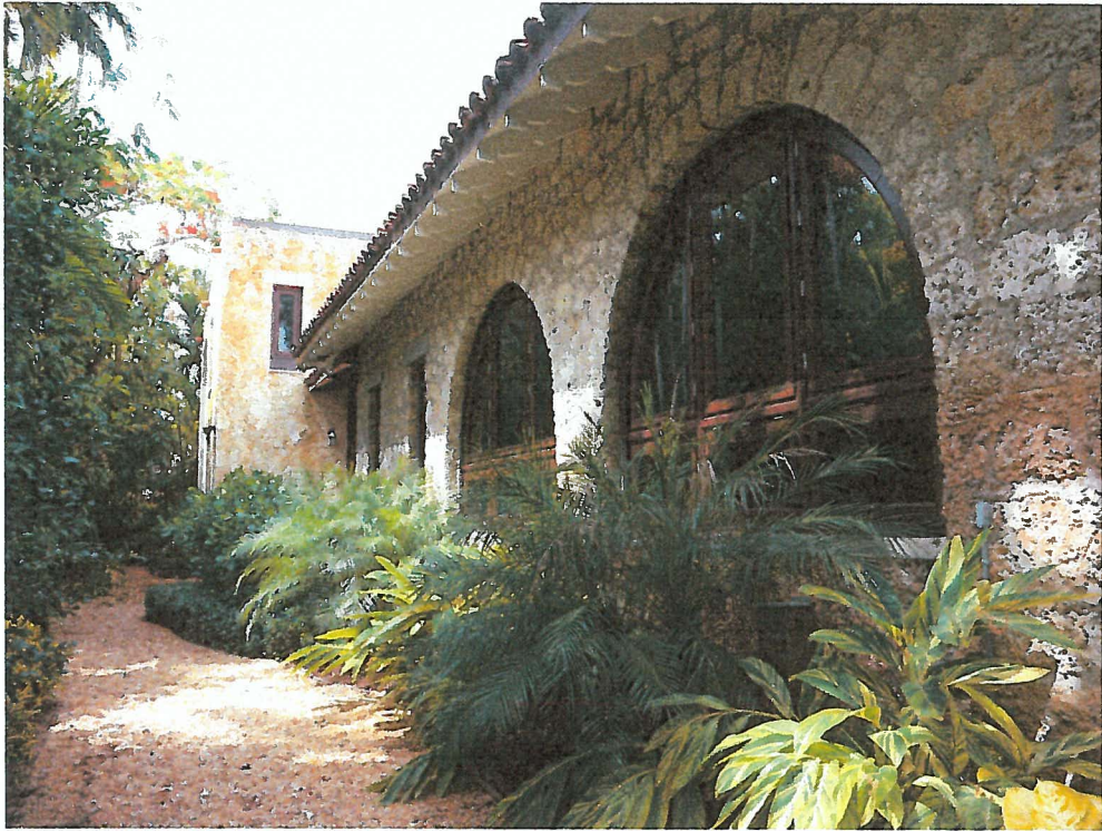
3. East Facade of Existing Residence
