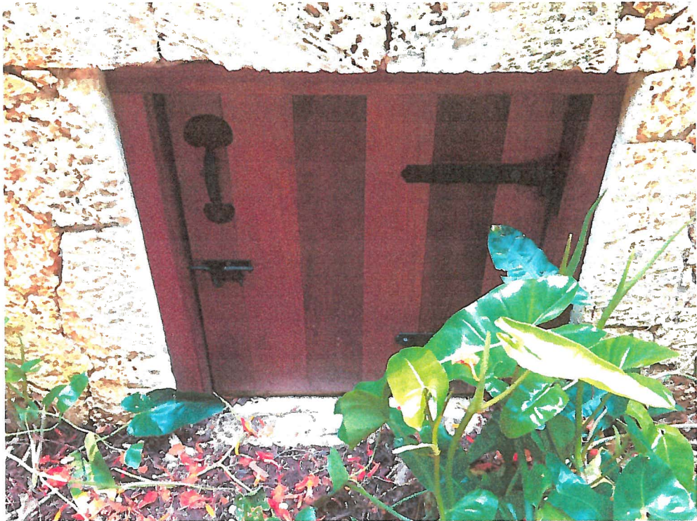
41. Existing Crawl Space
