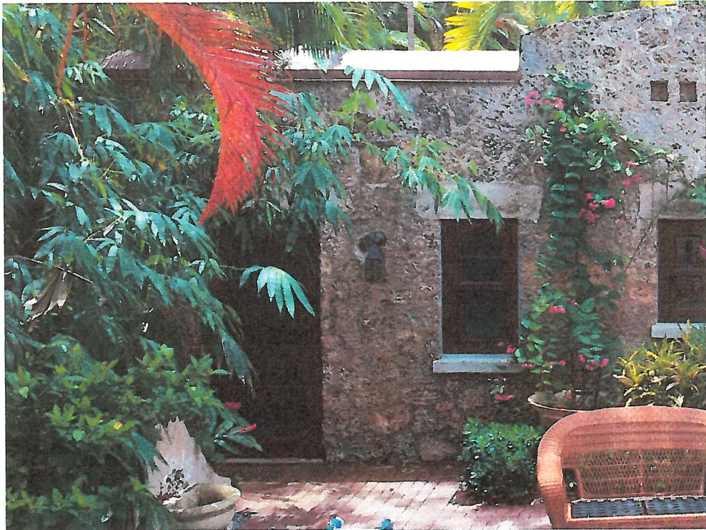
6. East facade of Existing Garage Detail
