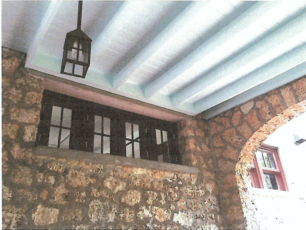
11. Exterior Carport at West
