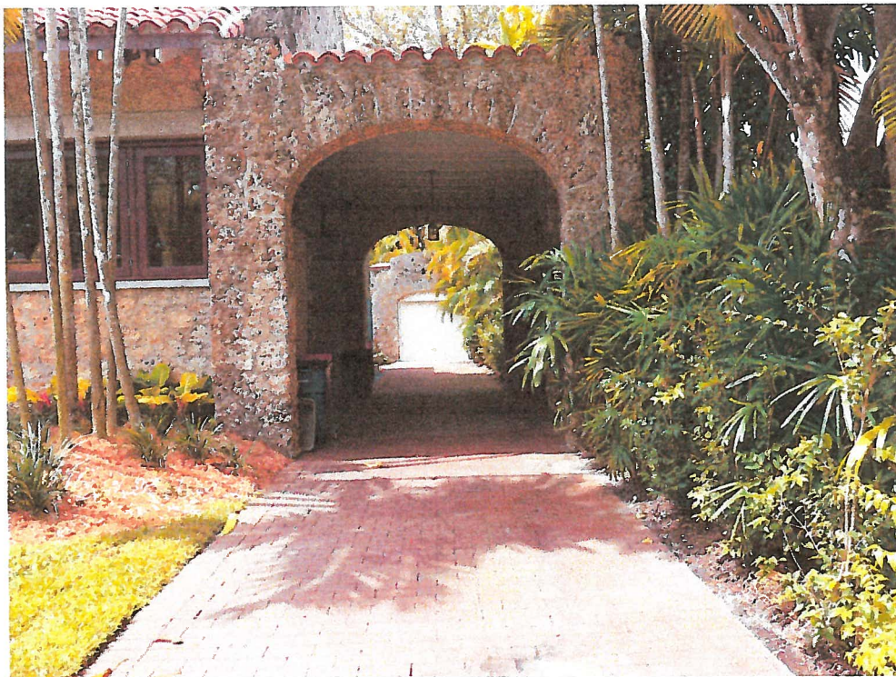
2. North Facade - Carport
