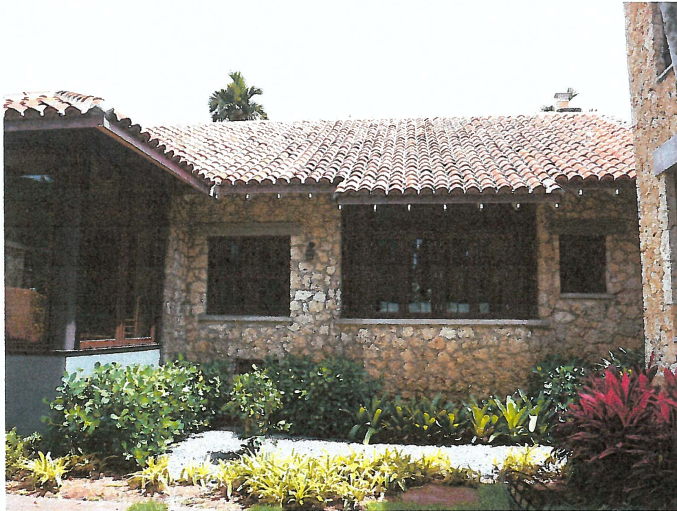
8. Southeast corner of Existing Residence
