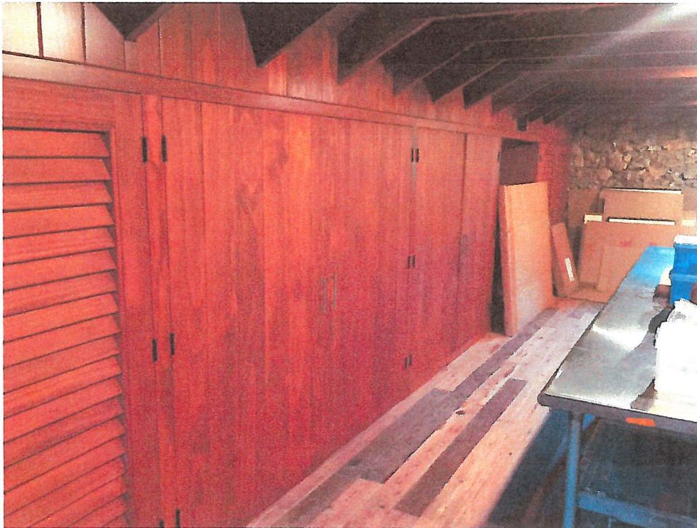
38. Attic Looking East
