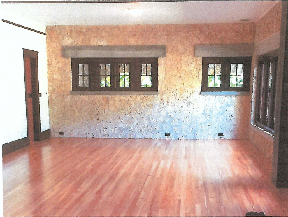
19. Dining Room Looking West
