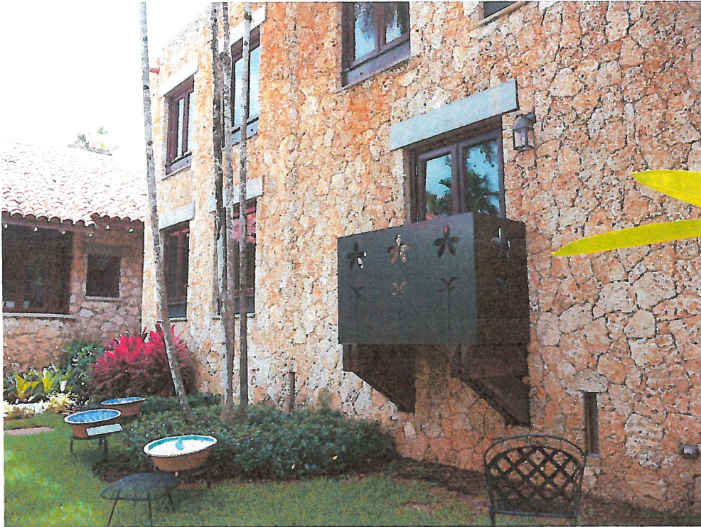
9. Existing Southeast Corner
