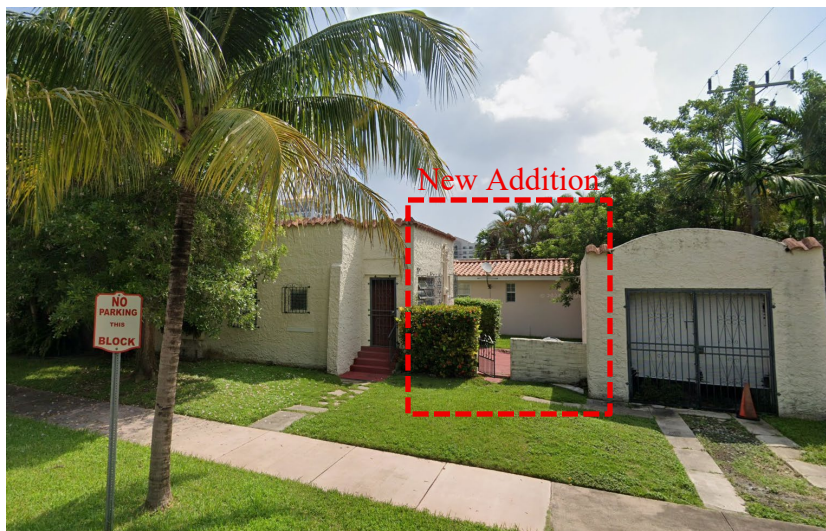
Figures 3: Existing Building Hernando Street | August 2024
