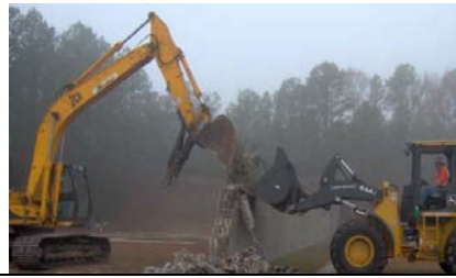
Demolition of brick wall between Firing Range Nos. 3 and 4
