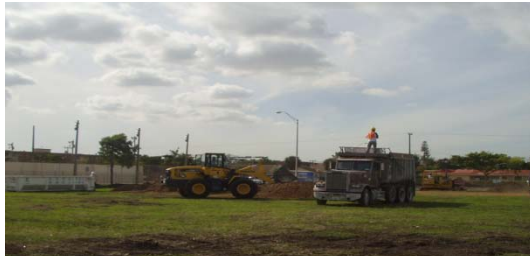
Loading AIS soil into trucks for disposal
