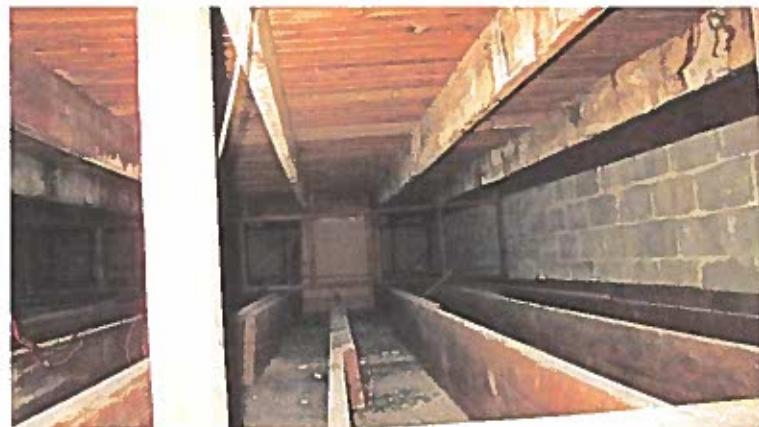
Photograph #8 of wood structure at second floor roof.
