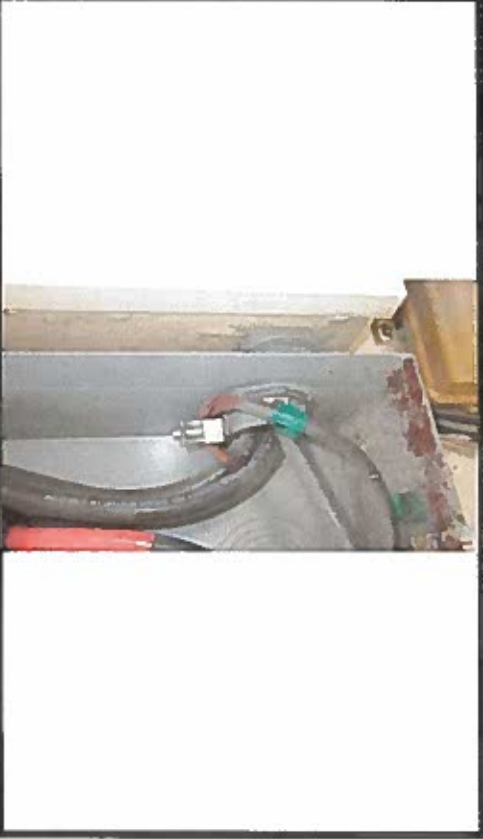
40-year Electrical Re-Certification Inspection - Photo 16
