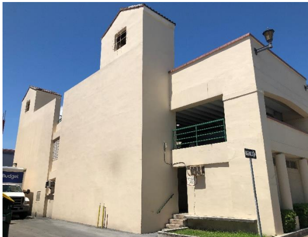
West and partial south elevations
