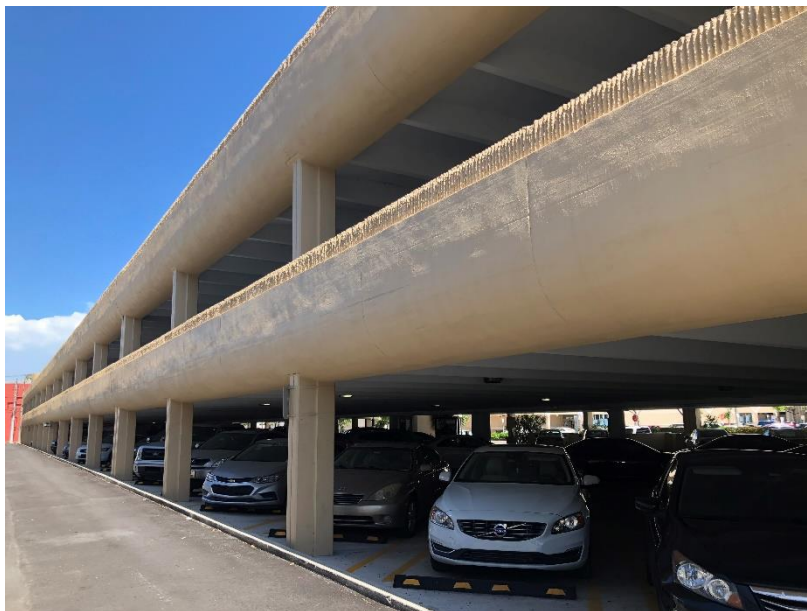
View of Parcel B looking southeasterly
