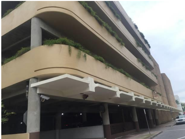
Looking southwest along north elevation.
