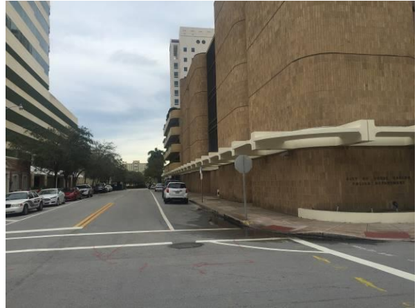
Looking east along north elevation and along Sevilla Avenue.
