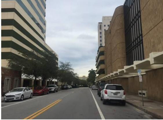
Looking east along Sevilla Avenue. Subject property at right.
