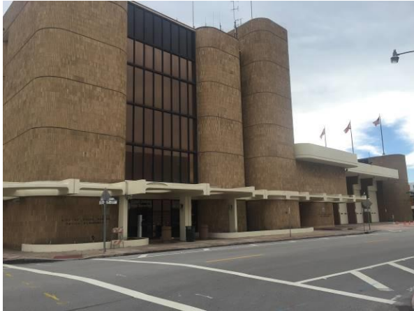
Looking southeast west elevation.
