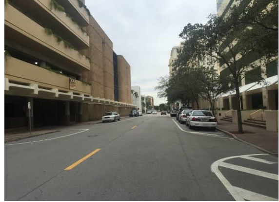
Looking west along Sevilla Avenue. Subject property at left.
