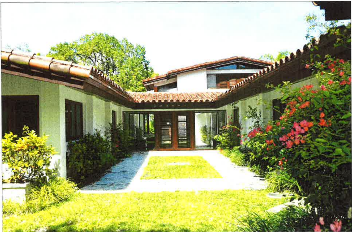
EXISTING RESIDENCE (CANDELA ADDITION)
