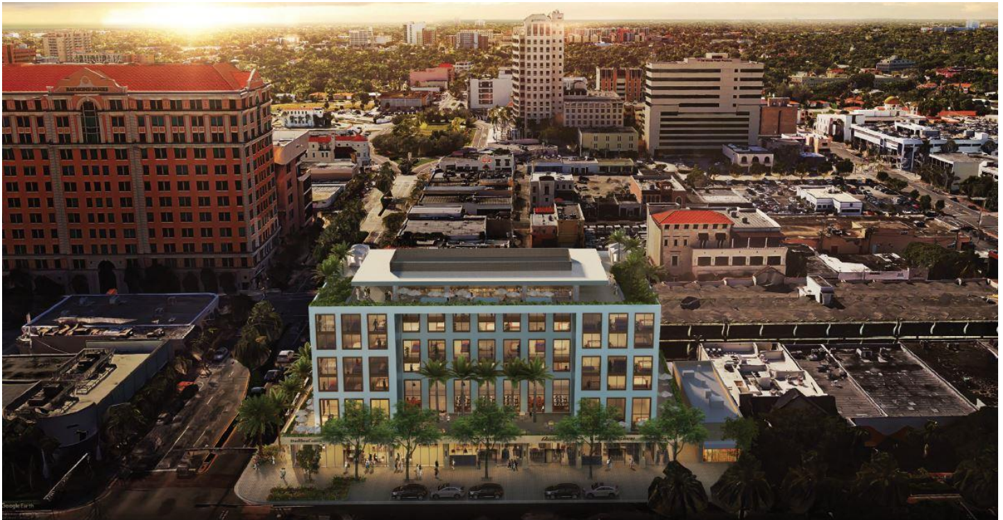
Proposed project and existing conditions
