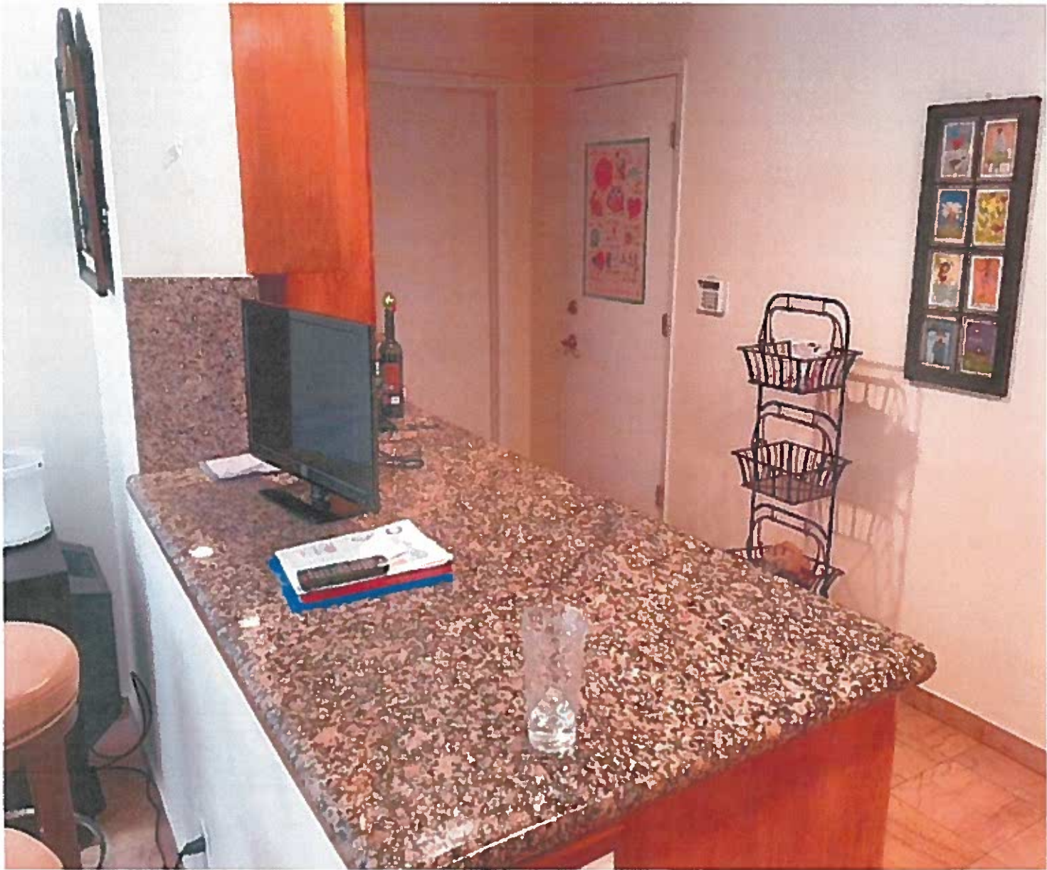
Kitchen, which remains as is. Glass on counter denotes location where plans show an "existing column." There is no column installed.
