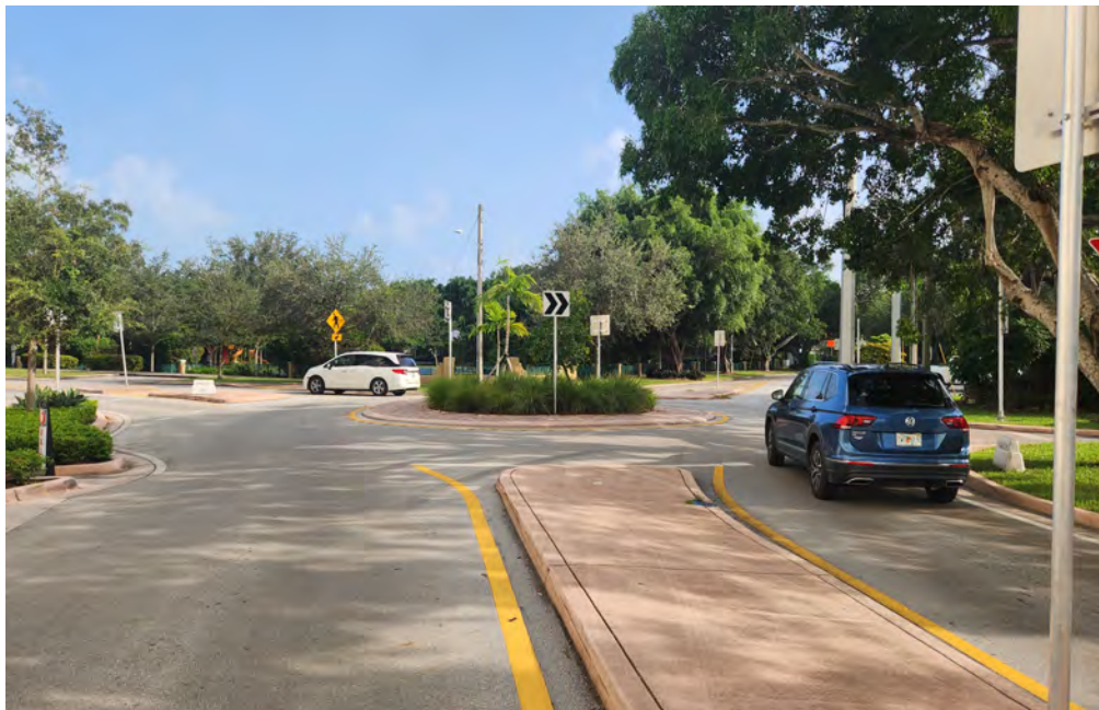
Roundabout at Caballero Boulevard and Hardee Road (Facing South): Moderate vehicular volume was observed along Caballero Boulevard (southbound approach)
