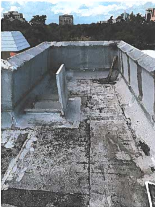
BUR Roof in Fair Condition
