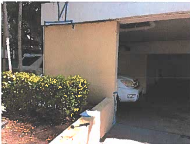
West Ground Floor Garage Entrance Beam Repair
