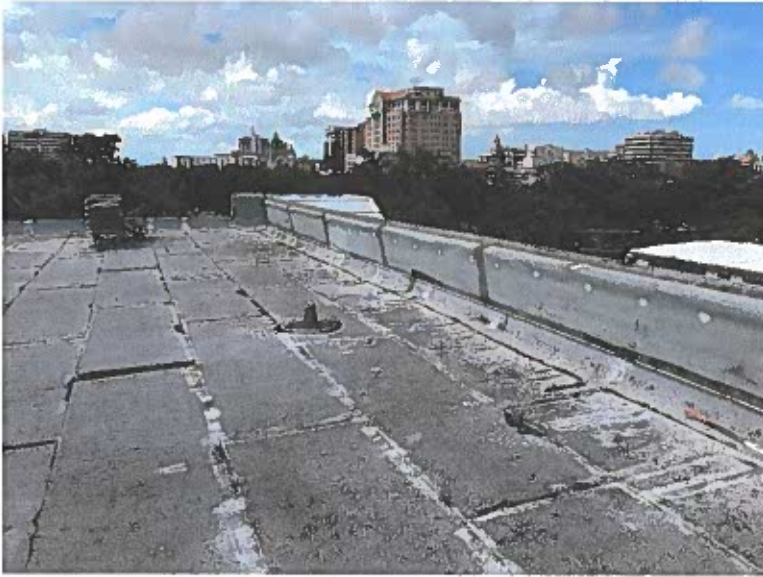
Roof & Parapet Wall
