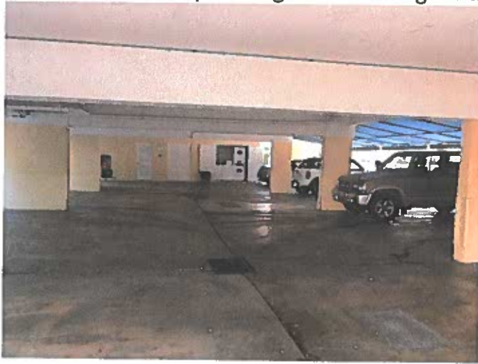
Garage at Ground Floor
