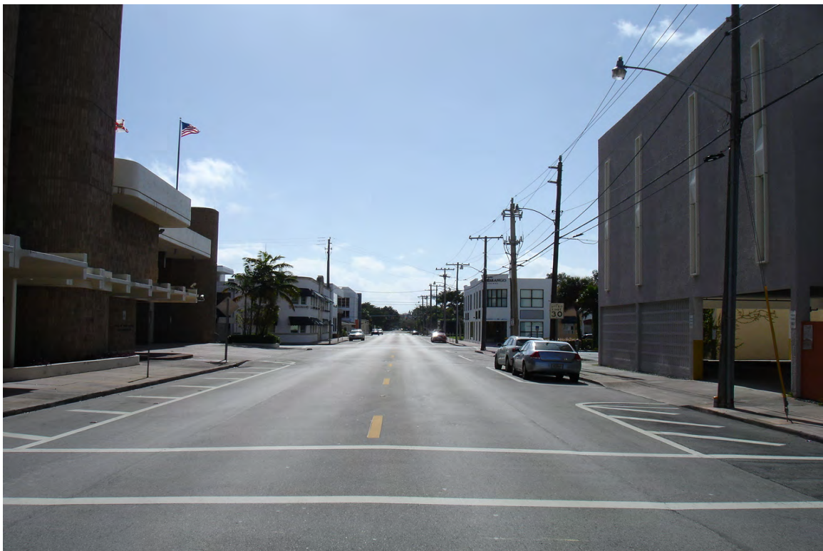
LOOKING SOUTHERLY ON SALZEDO STREET – SUBJECT TO LEFT
