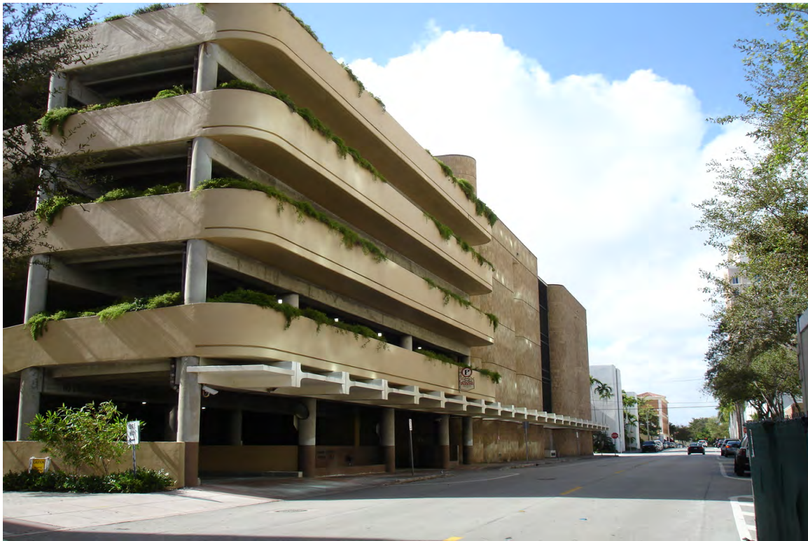
LOOKING SOUTHWESTERLY AT SUBJECT FROM SEVILLA AVENUE
