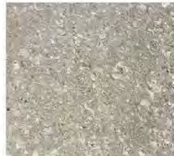
CONCRETE WITH EXPOSED COQUINA SHELL AGGREGATE
