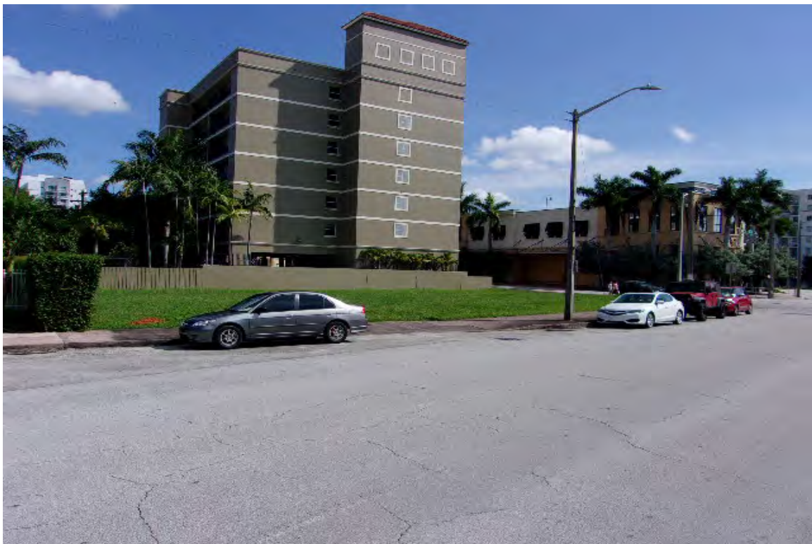
LOOKING NORTHEASTERLY AT SUBJECT FROM PONCE DE LEON BOULEVARD
