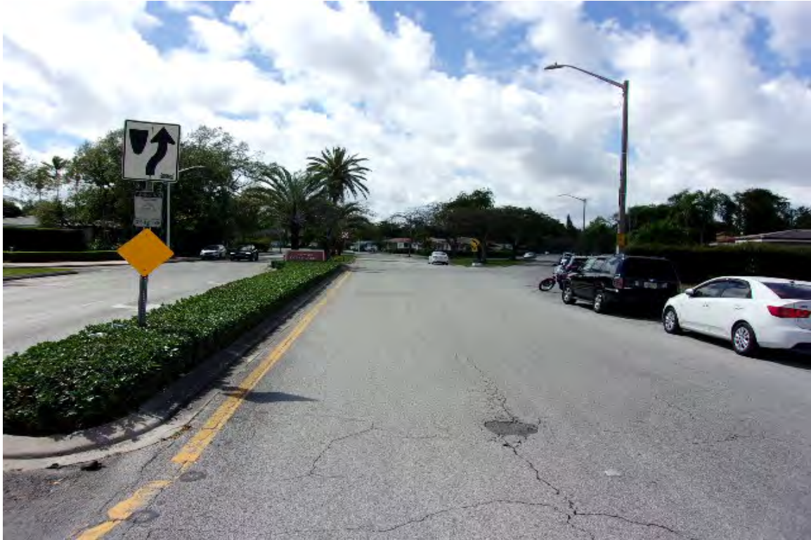
LOOKING EASTERLY ON PONCE DE LEON BOULEVARD – SUBJECT TO LEFT
