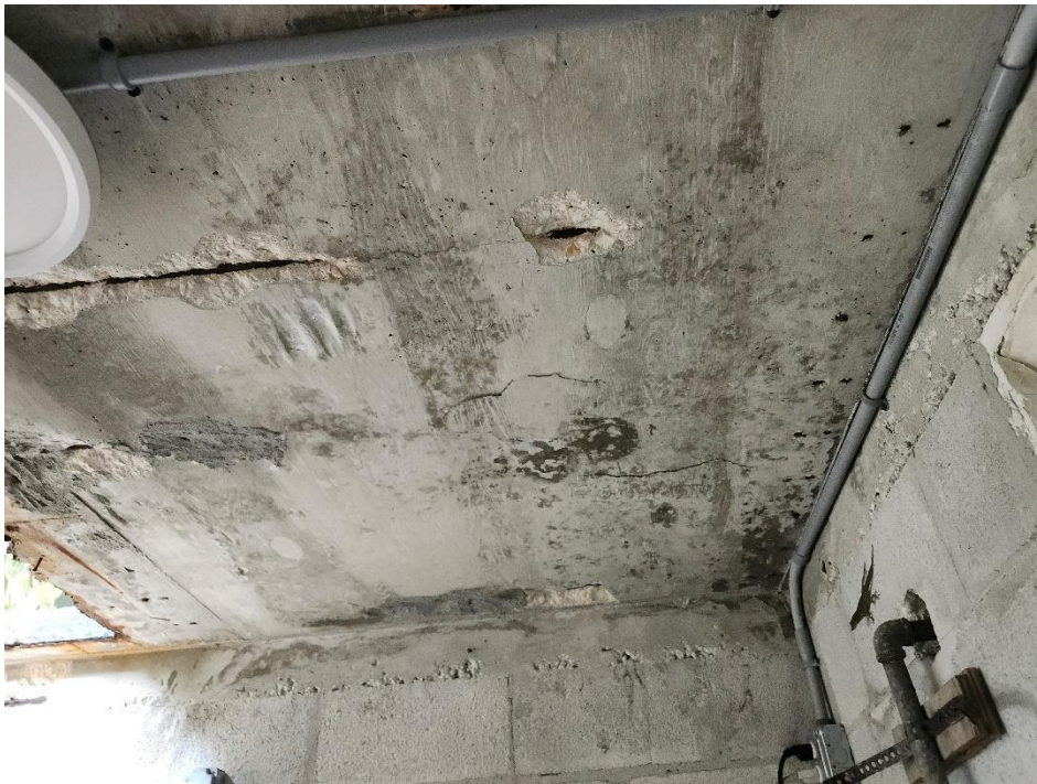
Pool room roof.
