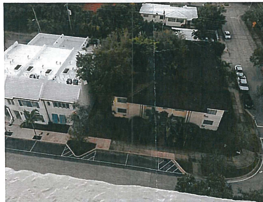
444 Valencia: project site aerial view
