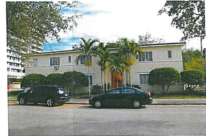
Project Site: view from Hernando Street
