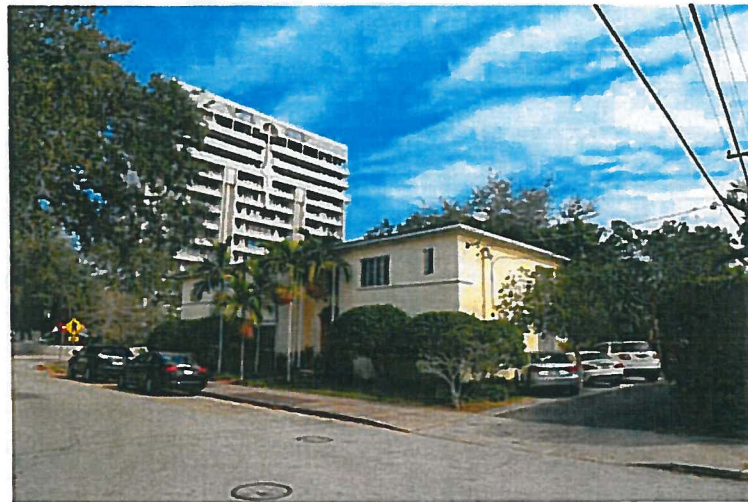
Project Site: view from Hernando Street
